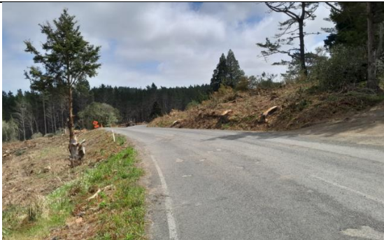
Kaitaia Awaroa Road Rehabilitation
