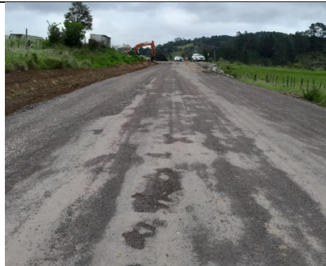
Pipiwai Road Rehabilitation
