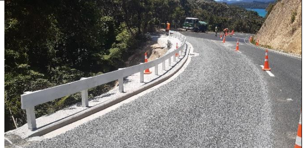
Manawaora Road Slip Repair with reinstated pavement and sight rail installed.
