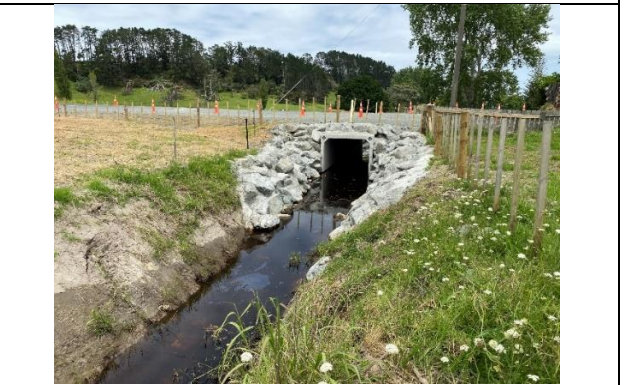
7/23/101 Quarry Road B13 Culvert Replacement
