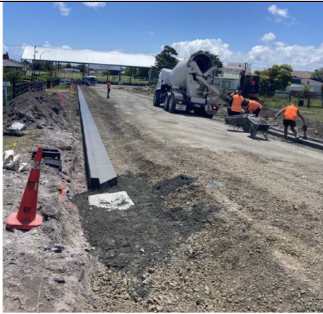
Sommerville Ave: Kerb and Channel, Urban Stormwater Replacement/ Road Rehabilitation Project
