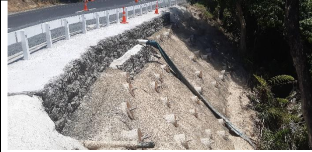
Manawaora Road Slip Repair with completed & hydroseeded soil nailed embankment.
