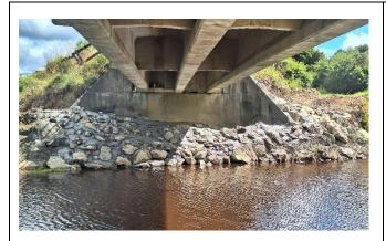
7/21/215 SP3 – Scour Protection Works at Pokapu Road Bridge T05 (North Abutment)
