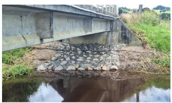
7/21/215 SP3 – Scour Protection Works at Pokapu Road Bridge T05 (South Abutment)
