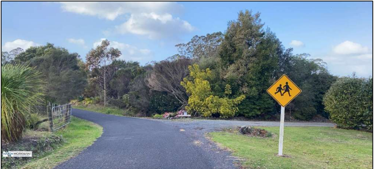
Chainage 120 - Entrance to no 12. 4.3m sealed carriageway width with vehicle crossing serving as a passing bay'
