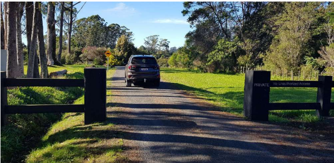
Entrance approx. 48m from Kerikeri Inlet Road. 2.5m lane width through gate, however there is adequate visibility on either side to see oncoming vehicles.
