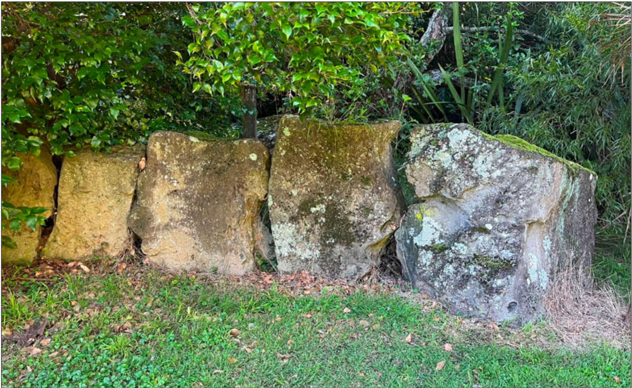
Figure 3: Site photograph of a basalt gravity wall upslope of the proposed building site.
