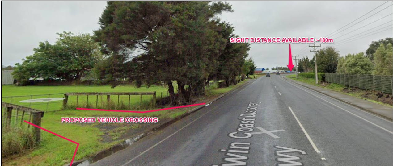
Figure 6: Annotated photo showing available sight distance from Vehicle Crossing 1 to the east
