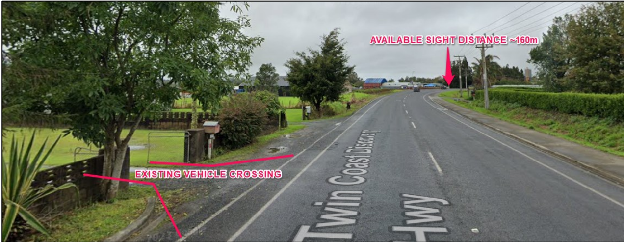
Figure 8: Annotated photo showing available sight distance from Vehicle Crossing 2 to the east
