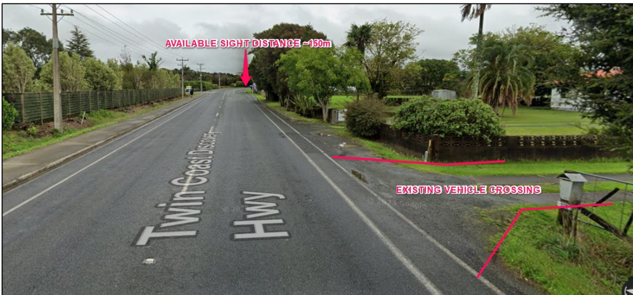
Figure 11: Annotated photo showing available sight distance from Vehicle Crossing 3 to the west
