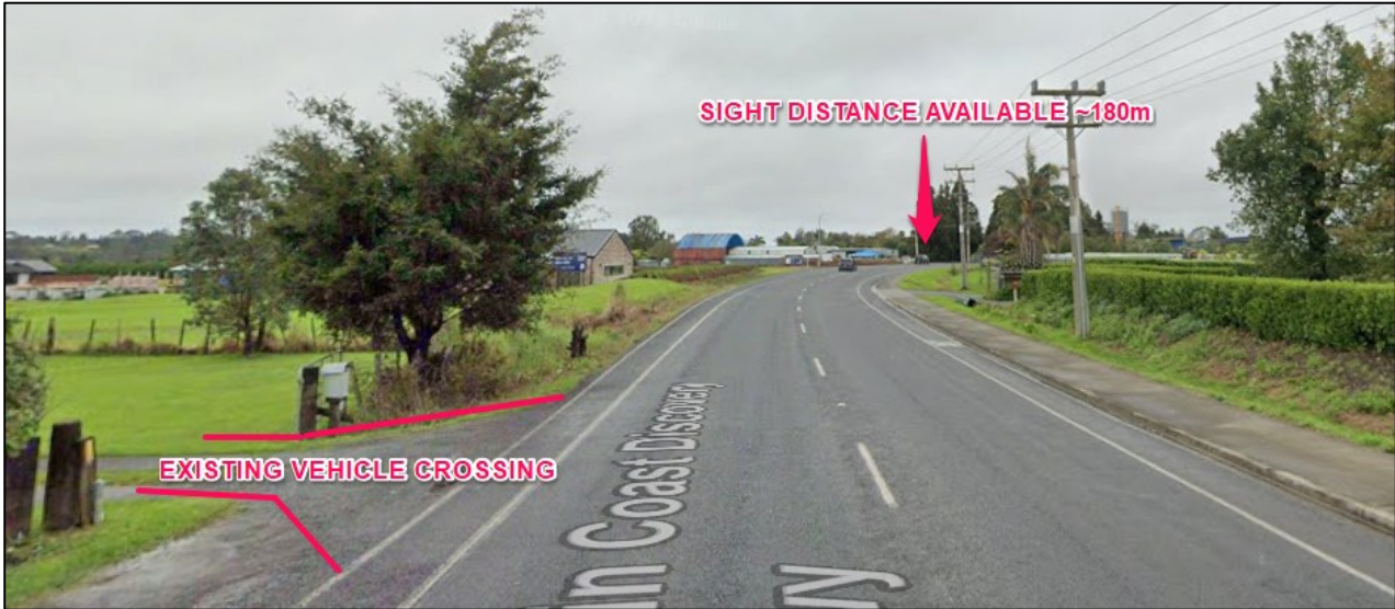
Figure 10: Annotated photo showing available sight distance from Vehicle Crossing 3 to the east
