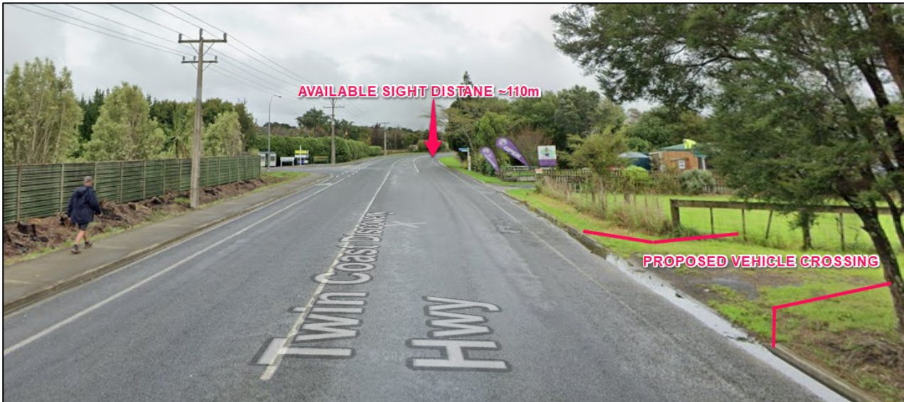
Figure 7: Annotated photo showing available sight distance from Vehicle Crossing 1 to the west
