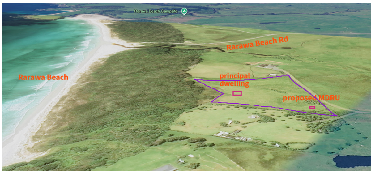
Fig.: Google Earth view showing Lot 3 and surrounding properties
