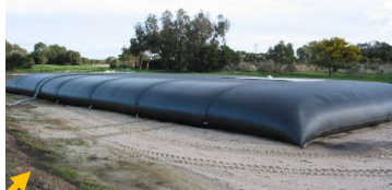
Solids dewatering geobags
