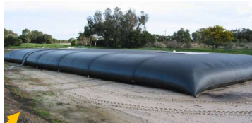
Solids dewatering geobags
