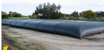
Solids dewatering geobags
