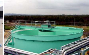
8 m diameter secondary clarifier
