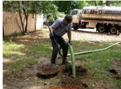
Septic tank pumpout
