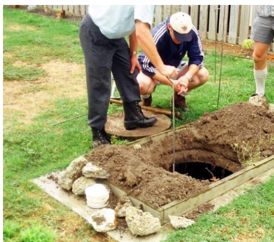
Checking scum and sludge levels in a septic tank
