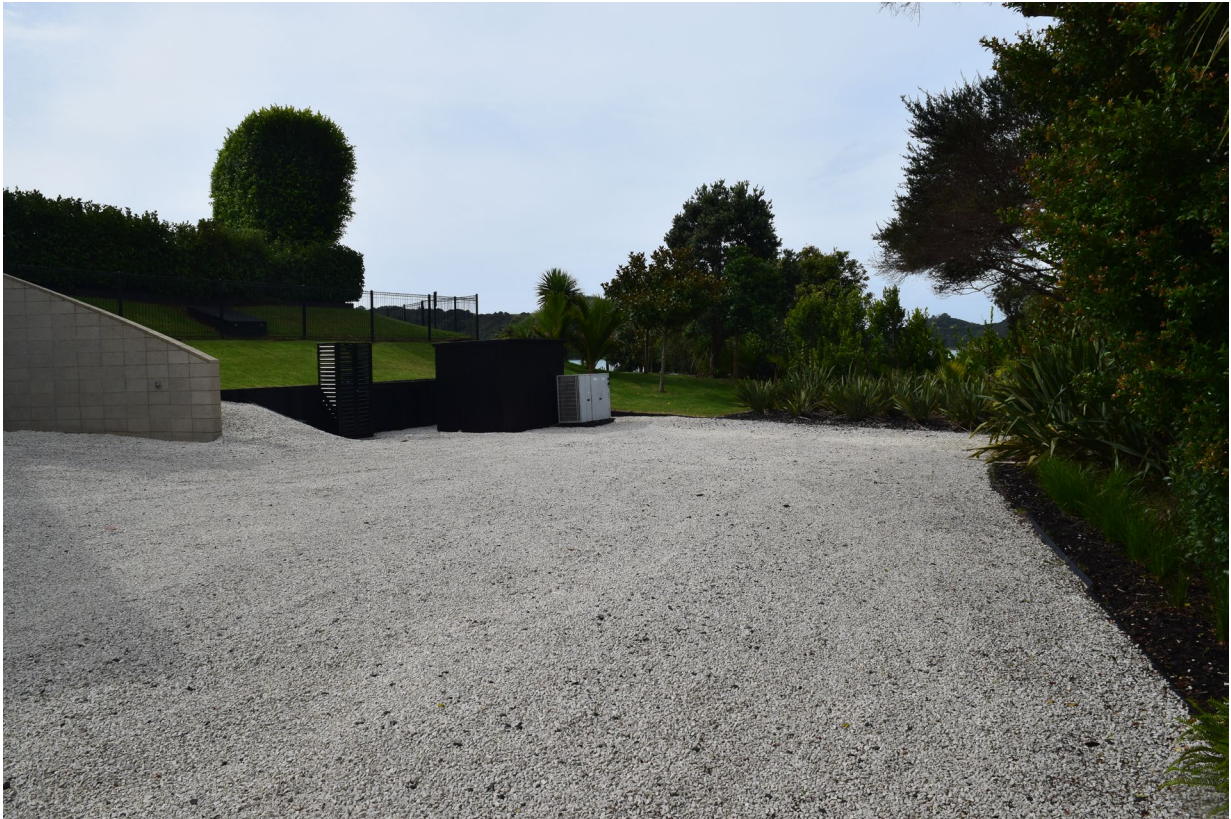
PLATE 1. THE AREA OF THE PROPOSED GARAGE, WALKWAY AND (part) DRIVEWAY EXTENSION (View to the north-east).
