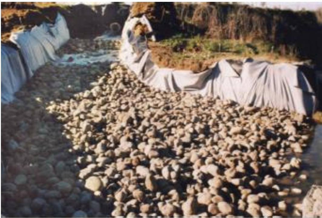
Figure 4 – Te Awamutu rock passage under construction (approximately year 2000)
