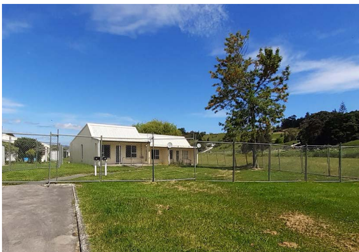
Units 13, 14 and 15 which are being demolished from 29 November 2021 due to structural issues
