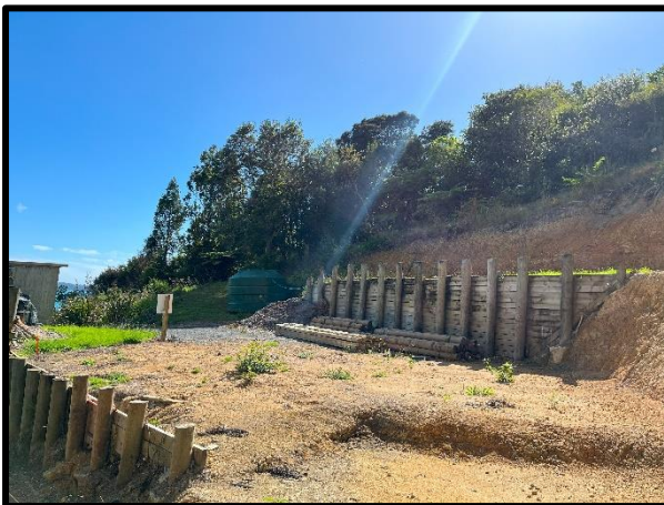
Figure 10: Building platform with two existing retaining walls. Cut face to the right of the image is proposed to be retained.
