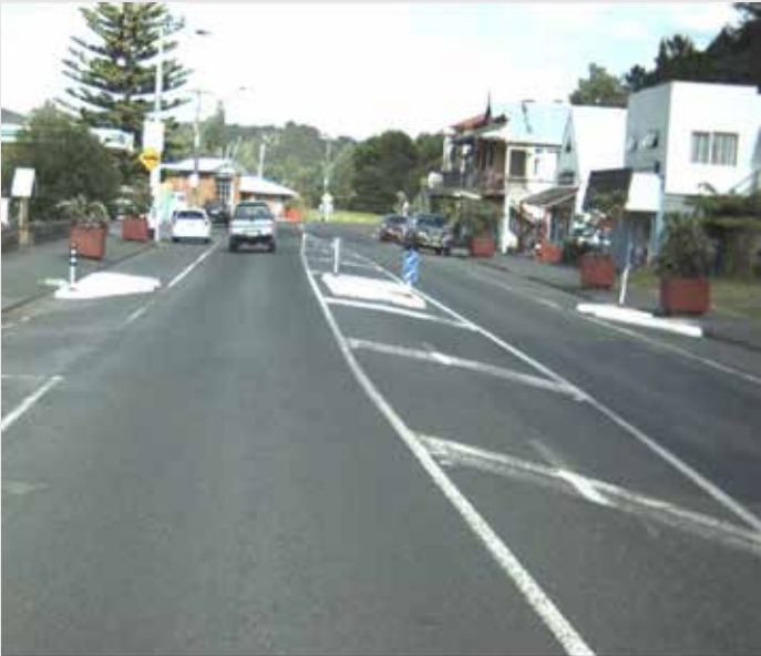
Recently constructed kerb buildouts and a pedestrian refuge in Kaeo create a safer place for people to cross the road.
