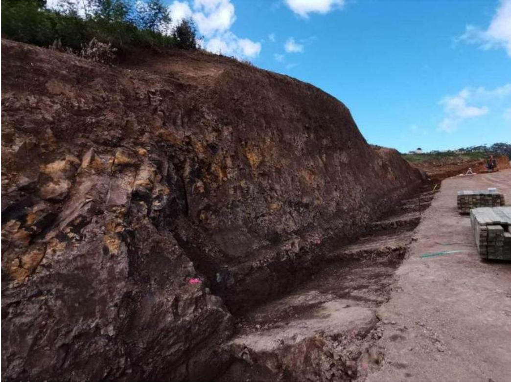
*Figure G – View north over excavation above Stage 5 access (photo taken during earthworks 2021). Weathering, Fracturing and faulting are evident in the underlying Basalt Rock*
