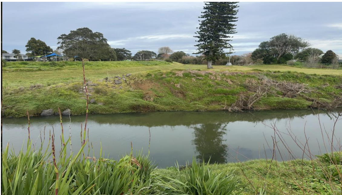
Figure 14 : Awanui River – Photo Facing West from top of Stop Bank Source Site Visit 17/09/2026
