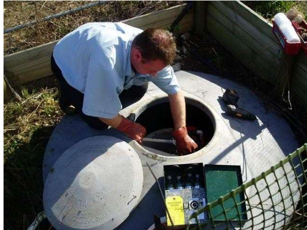
Servicing an advanced wastewater treatment unit
