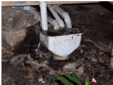
Backup to gully trap from clogged tank
