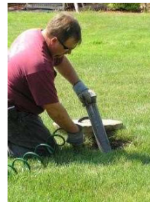
Lifting and hosing down effluent outlet filter
