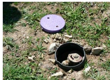
Automatic sequencing valve
