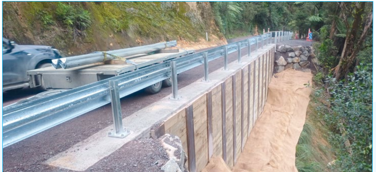
Slip repairs on Waikare Road included installation of 14 reinforced concrete piles supporting a 16m retaining wall with timber lagging.
