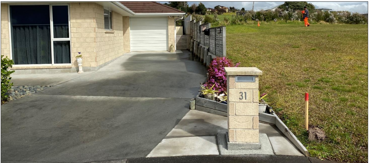
Figure 5: Site Photo – Overlooking the Neighbouring Retaining Wall to The East of Site.
