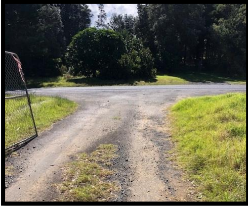
Figure 4: Vehicle Crossing from the site onto Far North Road.
