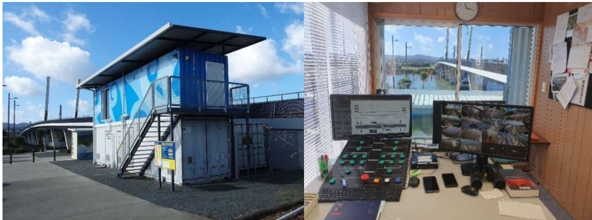
Figure 1-6: Bridge Control Room
