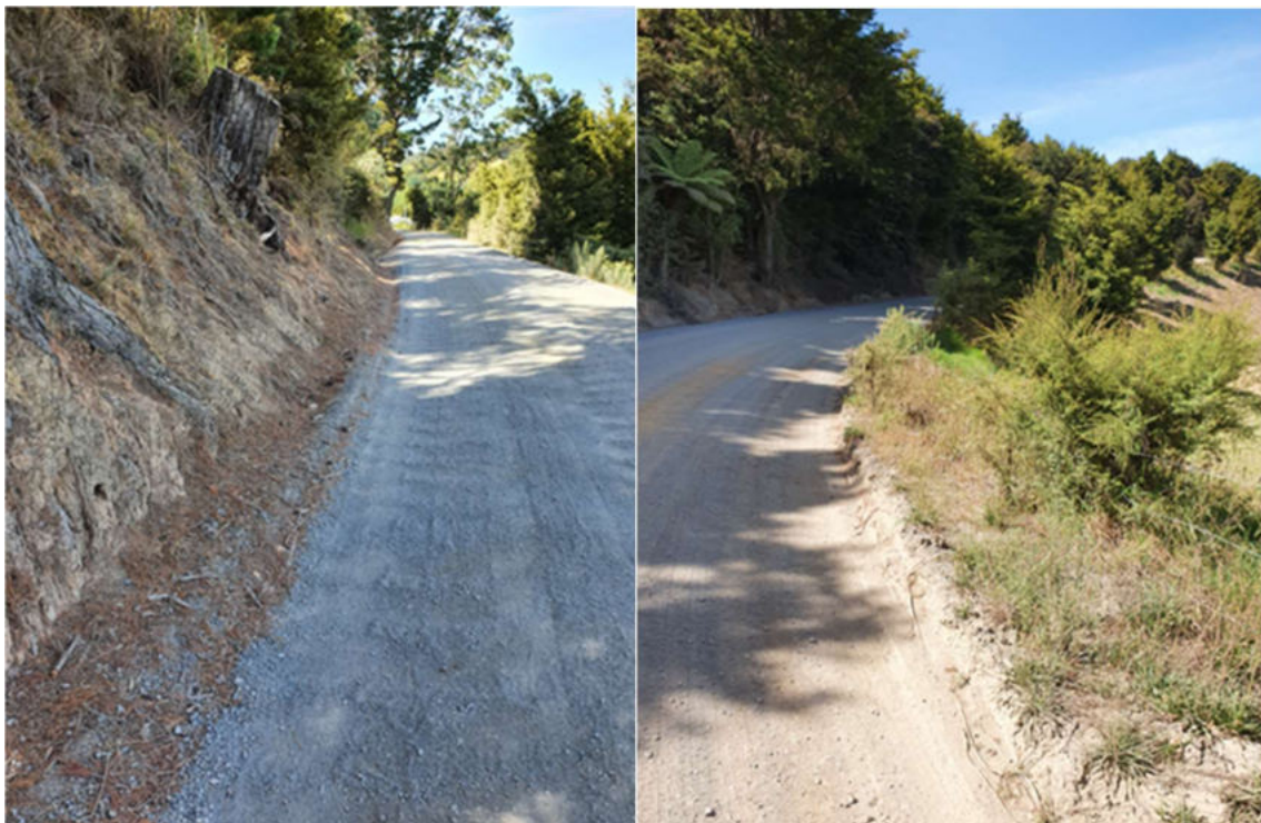
Figure 3-1: Inadequate watertables
