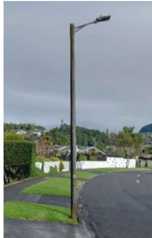
Figure 1-3: RCA owned concrete streetlight pole
