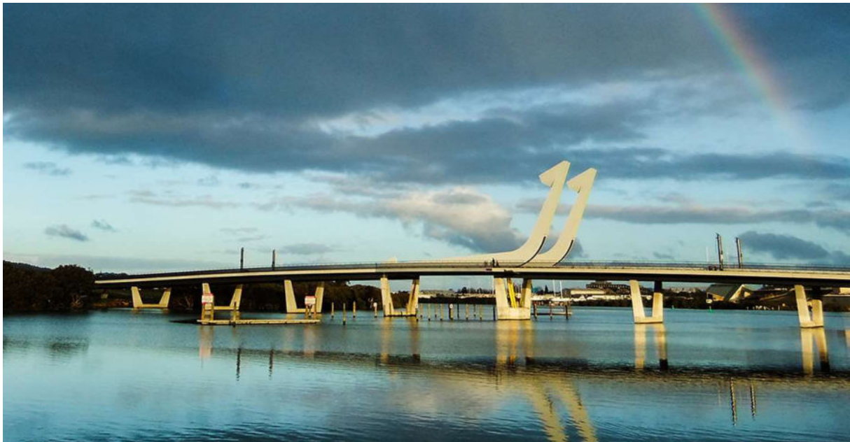
Figure 1-2: Te Matua ā Pohe bridge
