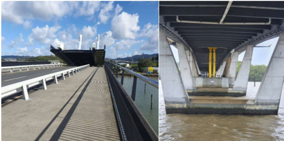
Figure 1-4: - Bascule lifting and Hydraulic RAMs at W1
