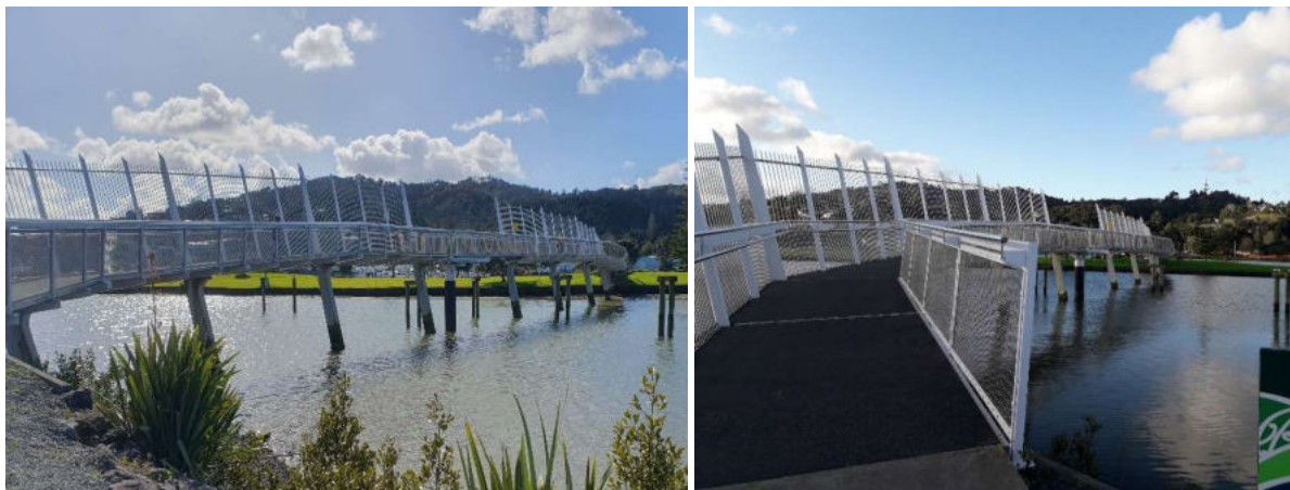
Figure 1-5: Kotuitui Whitinga Pedestrian Bridge
