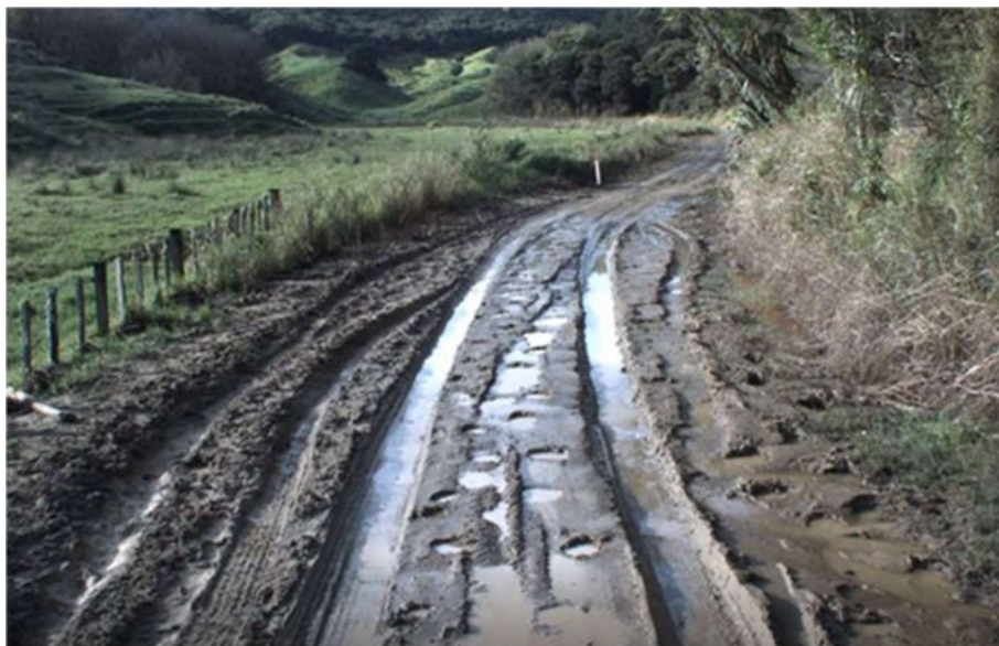
Figure 3-2: Inadequate watertables
