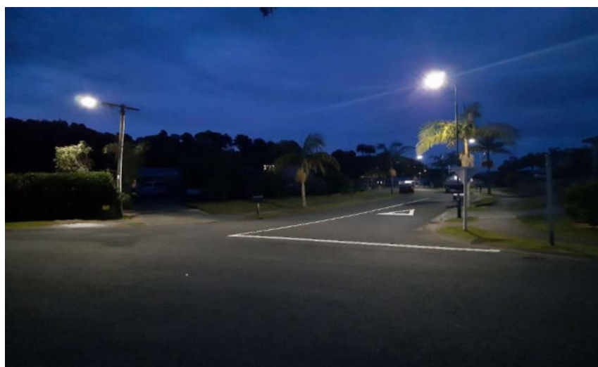
Figure 1-8: LED intersection lighting - Category P Road
