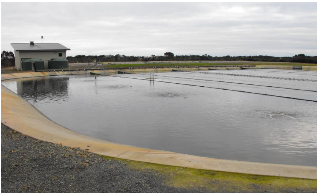
Figure 3.6 Photo of Pond 1 - note bubbles from airdisks and lines of aqua mats Ultraviolet (UV) Treatment
