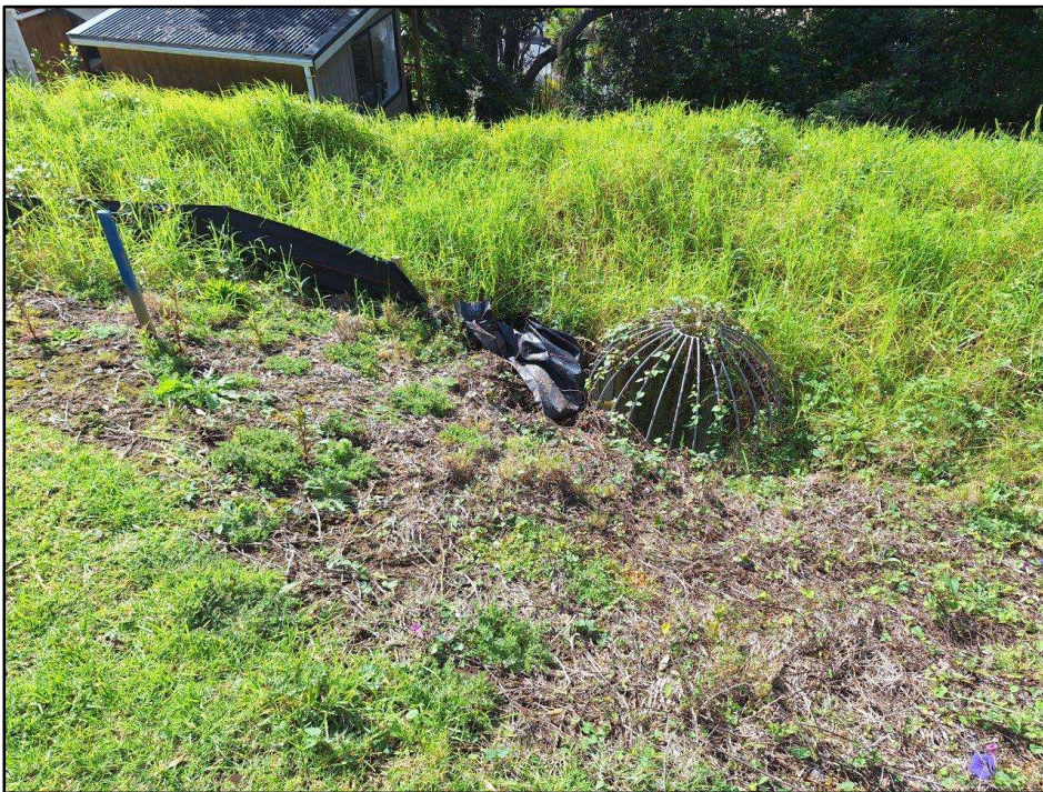
Photograph 4 – Stormwater scruffy dome manhole cover located on the southeast corner of the property.
