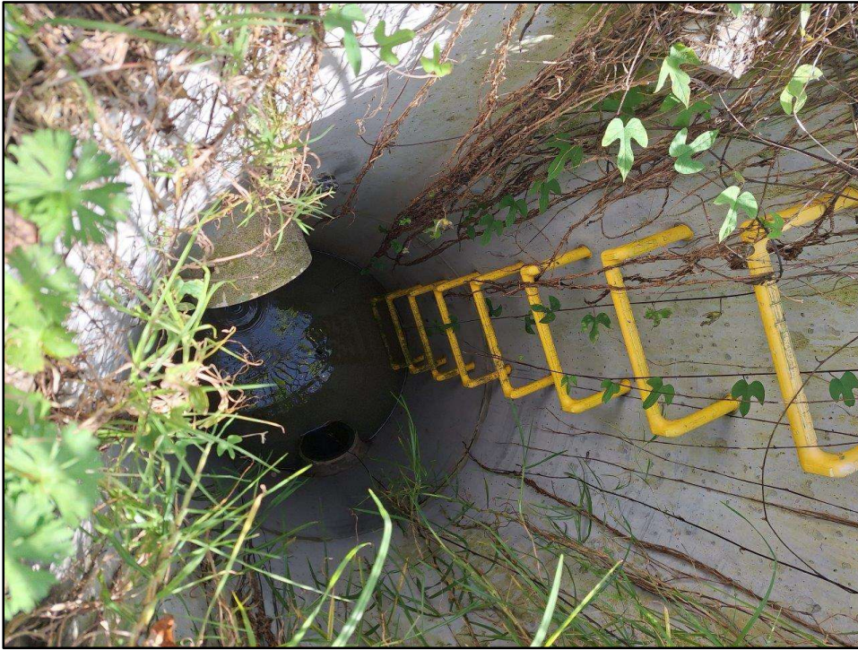
Photograph 5 – Stormwater manhole configuration located at the southeast corner of the site. A 150 mm PVC lot connection is visible in the photograph at the top right corner.
