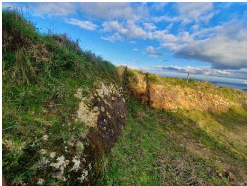
Photo 3: Shallow rock encountered in the existing earthworks cut at the location of the future parking.
