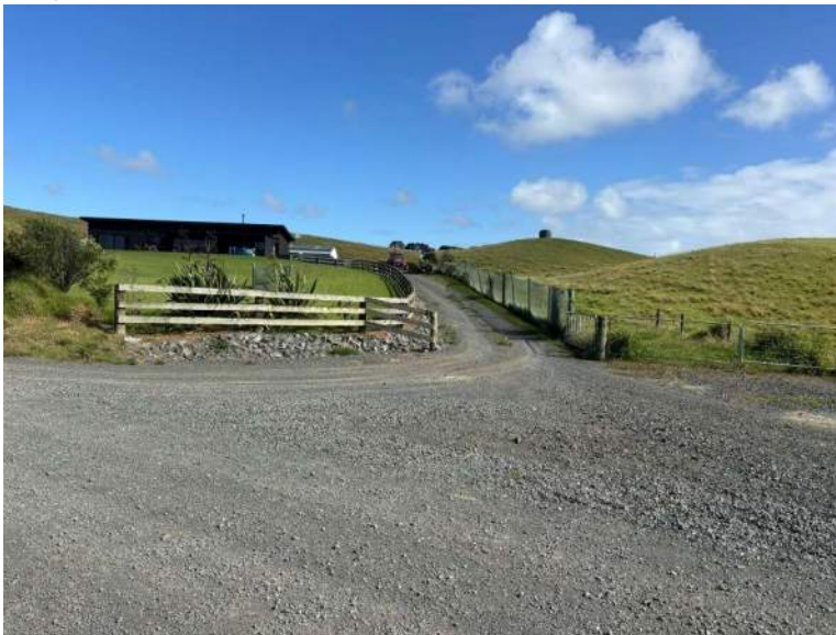
Figure 7- Lot 2 existing accessway
