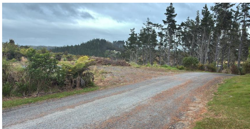
Figure 4 - New driveway into building platform off ROW
