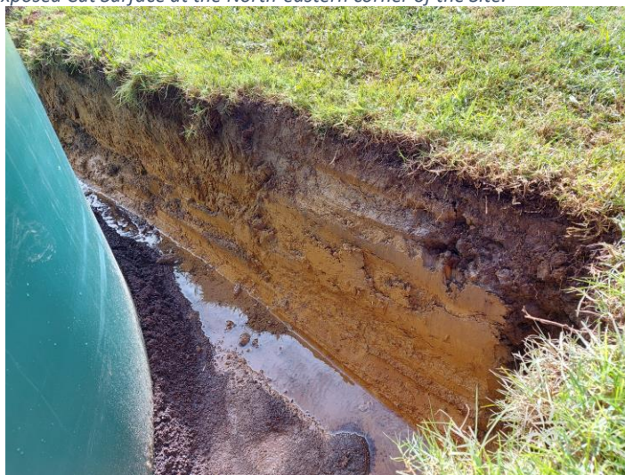
Figure 5: Observed Exposed Cut Surface at the North-eastern corner of the Site.
