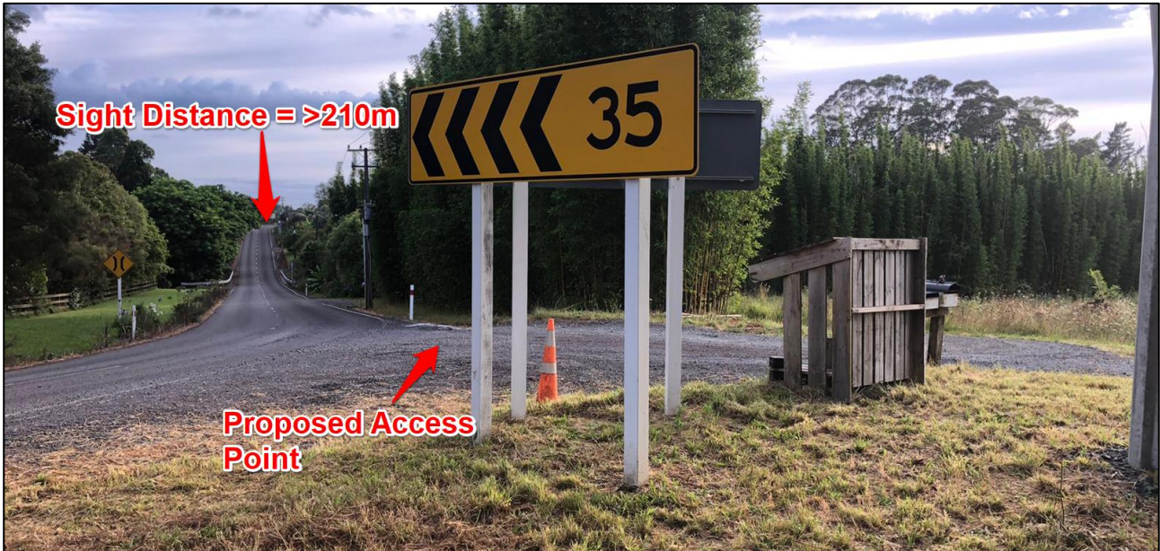
Figure 15: Proposed Vehicle Crossing Location on Koropewa Road Facing Northeast, >210m Sight Distance Available.
