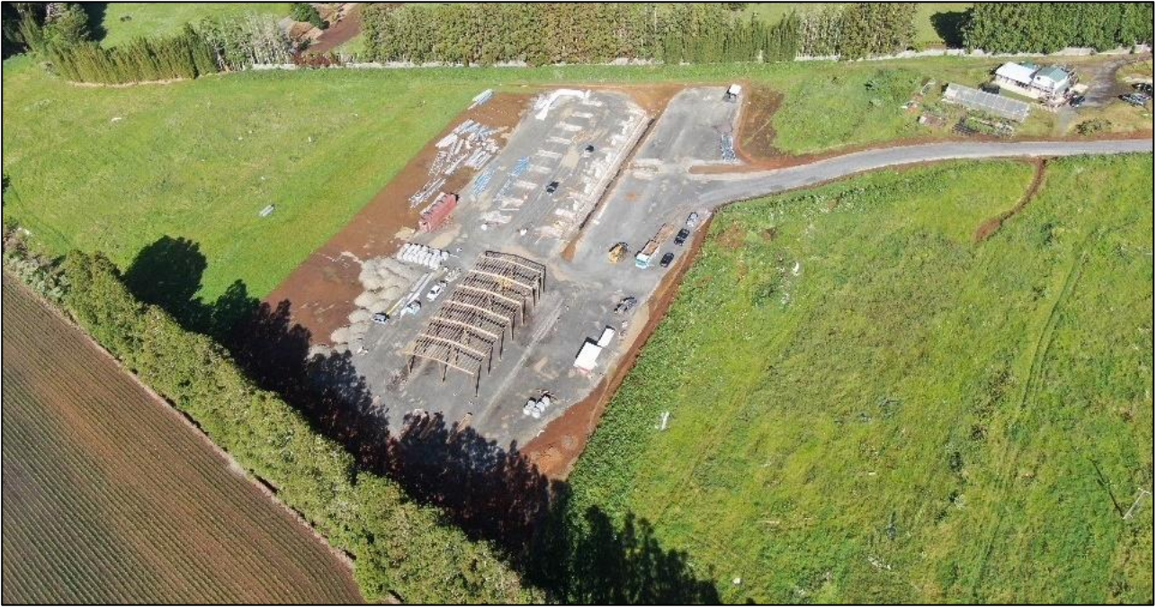
Figure 6: Drone aerial photo of the existing dwelling and factory in construction.
