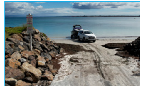
The Rangiputa boat ramp has been upgraded.
