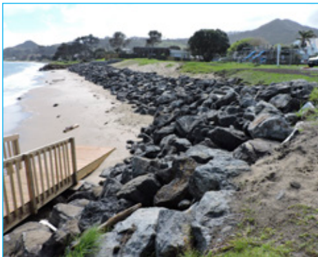
The new seawall and beach ramp are now in place at Freese Park Reserve, Ōmāpere.
