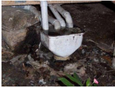
Backup to gully trap from clogged tank
