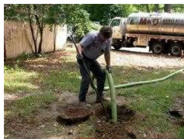
Septic tank pumpout
