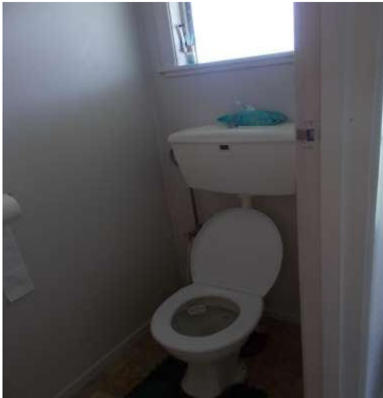
WC. Surface sider entry, vinyl floor, Ceramic bowl, Good condition, older dux cistern..
