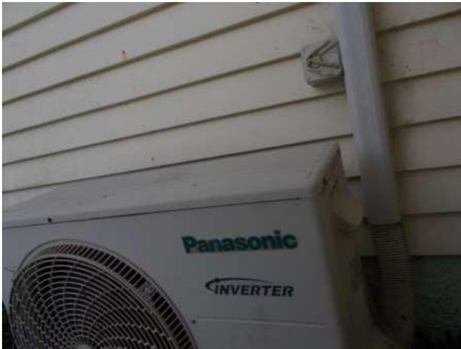
Heat Pumps: Panasonic CU series inverters (2)
