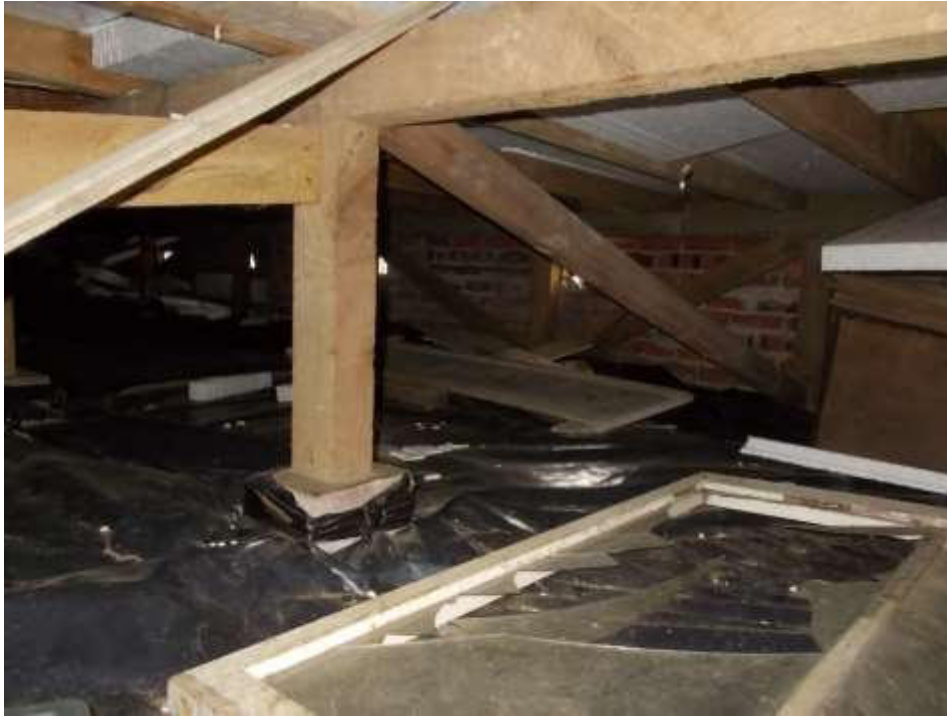
Subfloor: 90x90 bearers on 100x100 piles, diagonally braced with a brick masonry subfloor cladding
