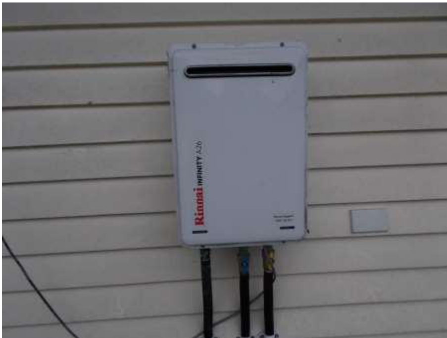
Hot water: Rinnai infinity A26 series on demand caliphont. This unit appears to be quite new.
