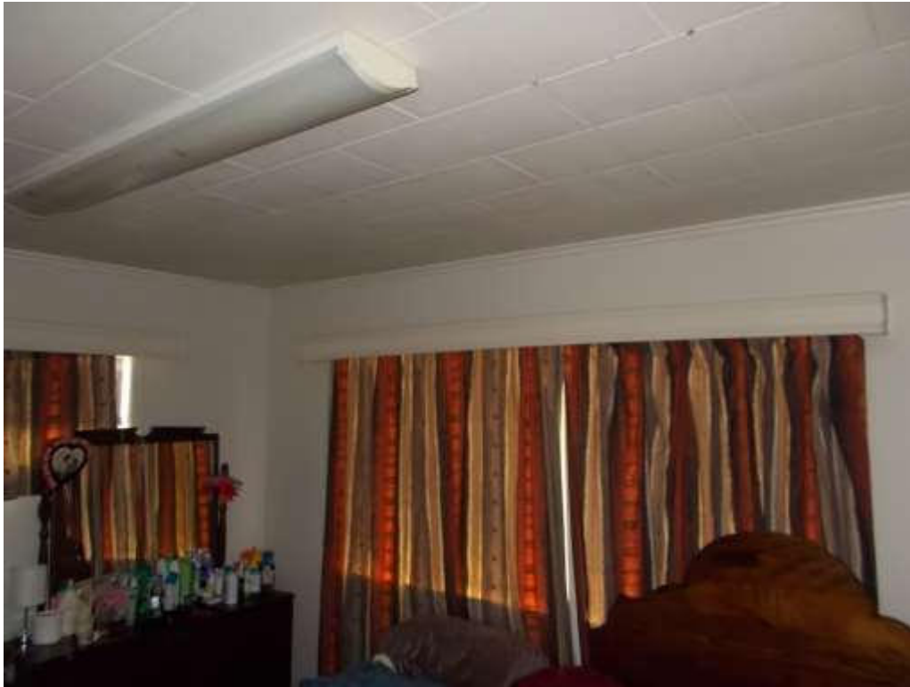
Bdr 1: Clean, 12mm pinex tile ceiling, fixtures appear ok.
