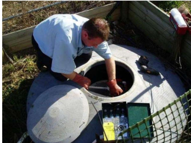
Servicing an advanced wastewater treatment unit
