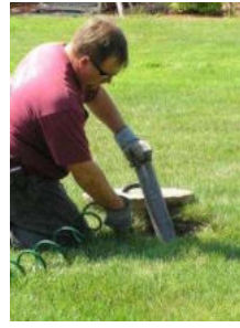
Lifting and hosing down effluent outlet filter
