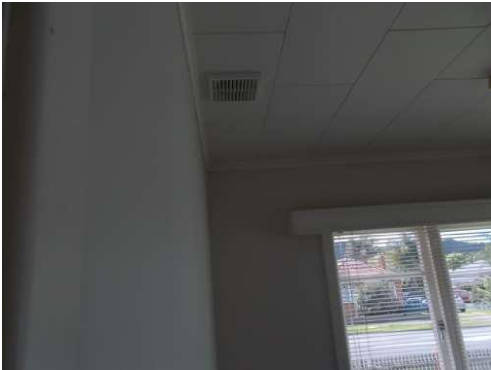
Bdr3: DVS Venting system to all bedrooms, standard scotia finished to ceiling junction
