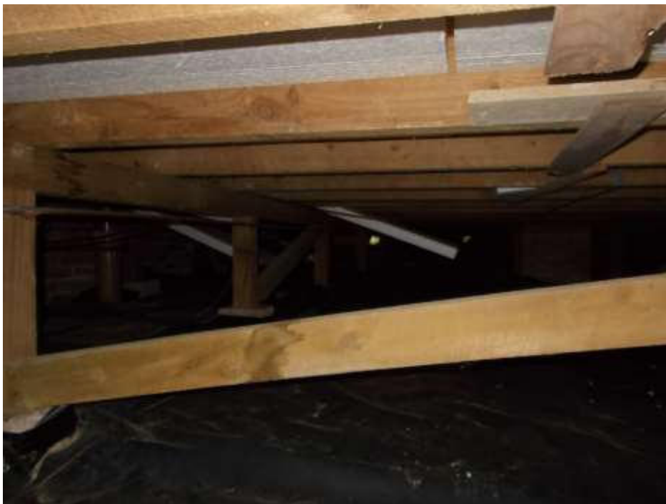
Floor: Diagonal bracing. Tongue and groove flooring was checked in several locations and appears to be in quite good condition, suitable for polishing.
