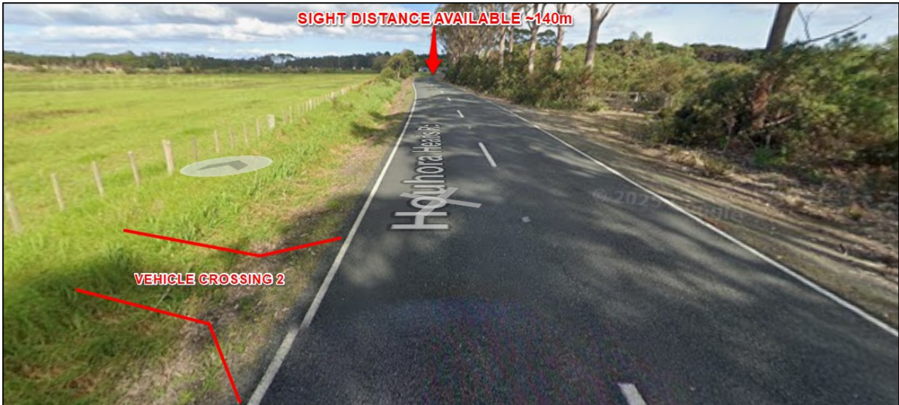
Figure 7: Annotated photo showing available sight distance from Vehicle Crossing 2 to the southwest
