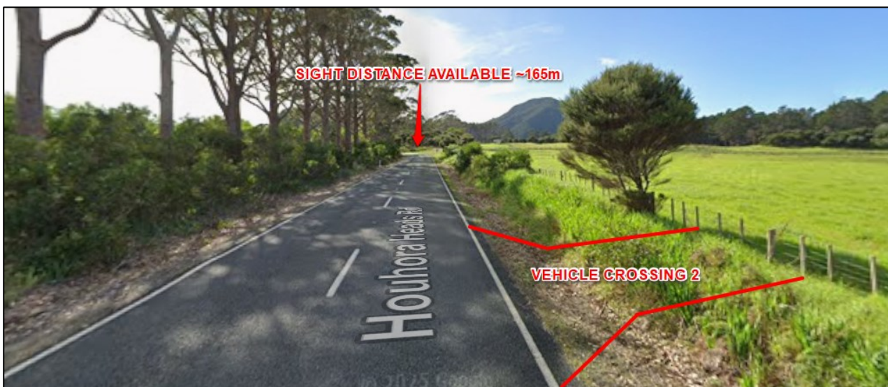
Figure 6: Annotated photo showing available sight distance from Vehicle Crossing 2 to the northeast
