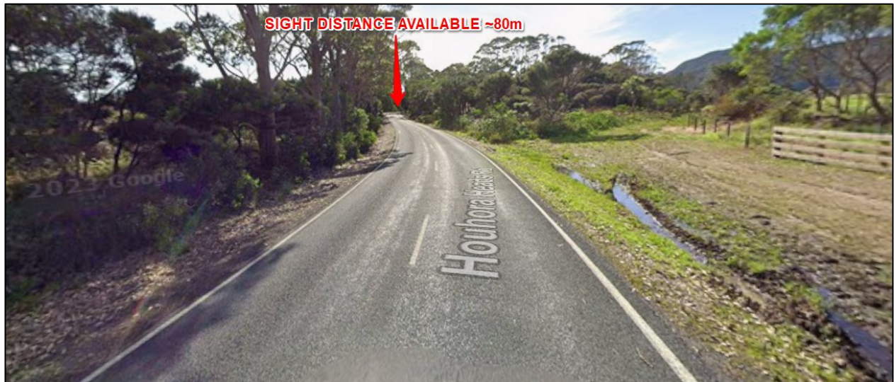
Figure 8: Annotated photo showing available sight distance from Vehicle Crossing 3 to the northeast
