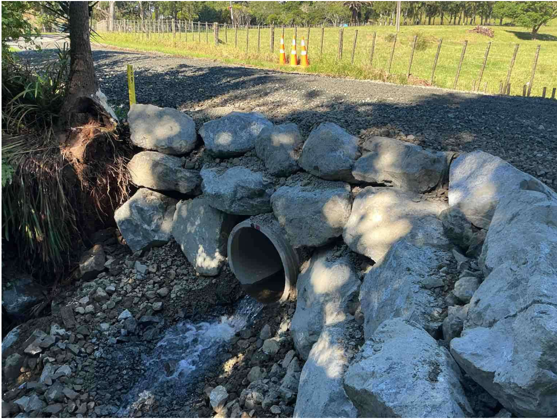
Kaiawe Rd – Storm Damage repair completed headwall
