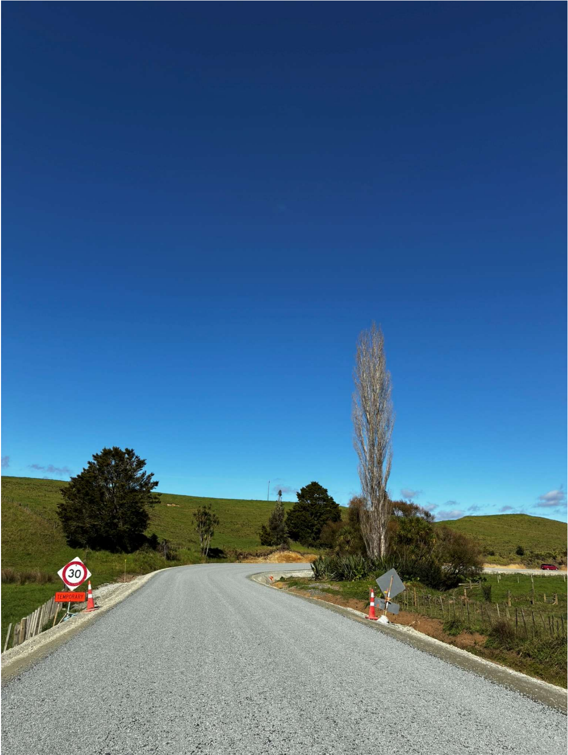
Fairburn Rd Rehab – New Seal
