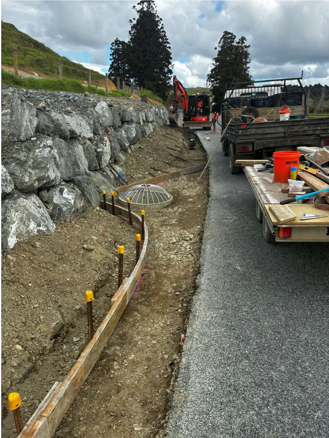
Fairburn Rd Rehab – Dish Channel Construction (Sweetwater Construction)
