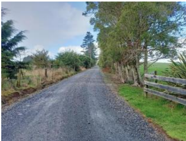
Figure 4: Existing driveway within site which will form ROW C.
