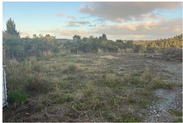
Figure 6 - Cleared building platform looking south
