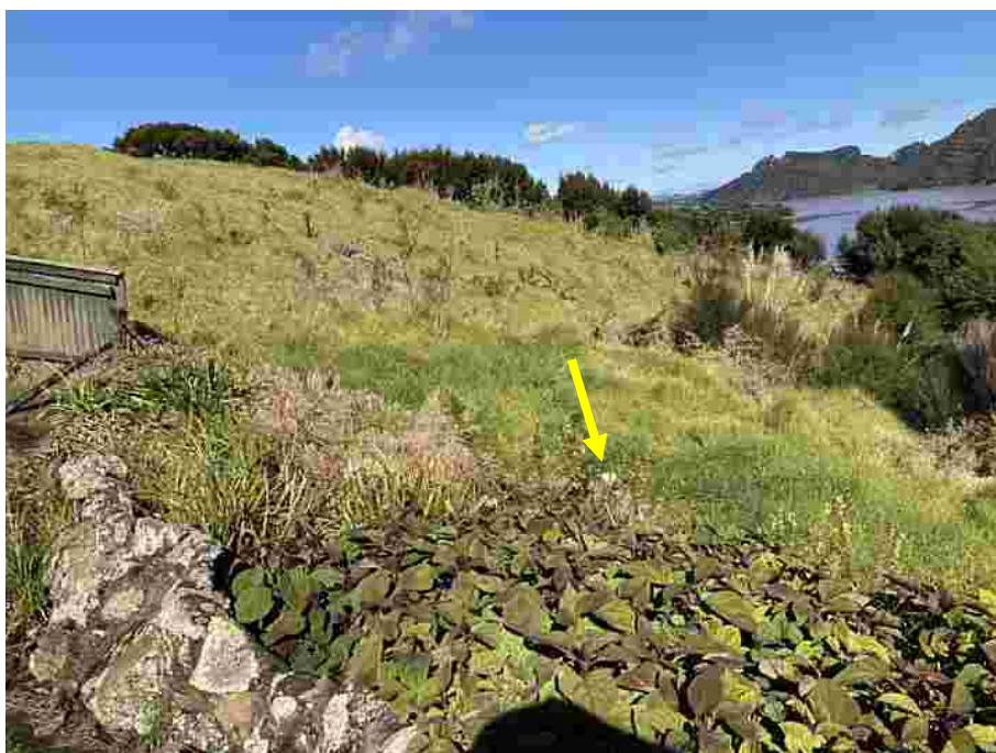
Figure 16:: Lot 2 inferred location of septic tank to boundary (looking south)
