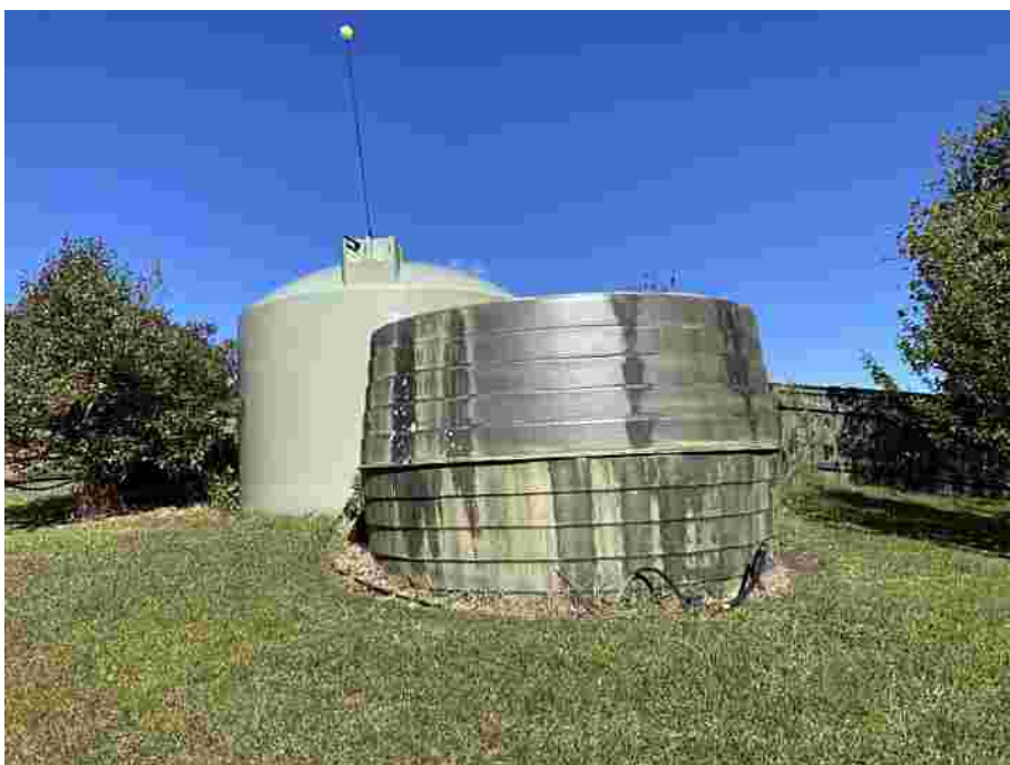
Figure 18: Lot 2 Water supply tank pumped from spring water (pump in foreground is redundant).
