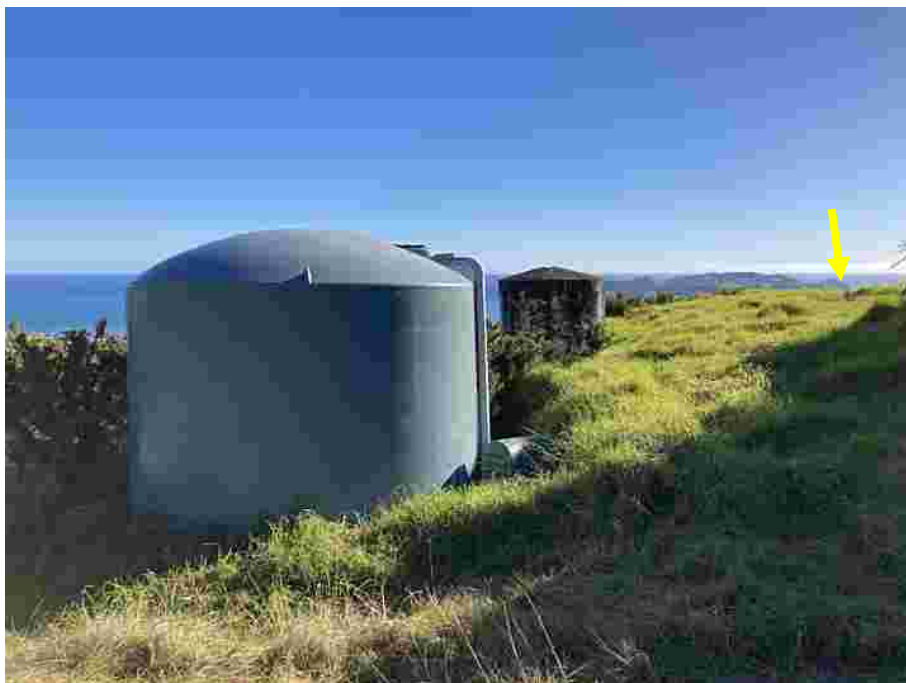
Figure 13: Lot 1 Rainwater tank and pump relative to septic tank in background
