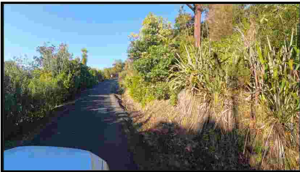
Figure 4 – Lower chip-sealed part of accessway
