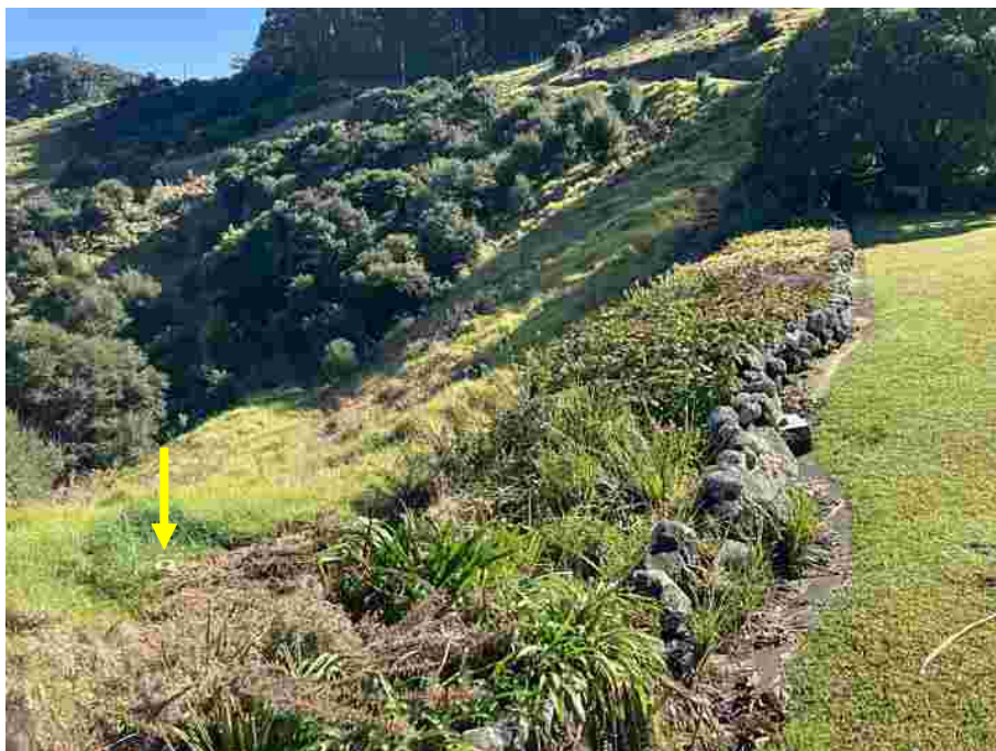
Figure 15: Lot 2 inferred location of septic tank to boundary (looking north)
