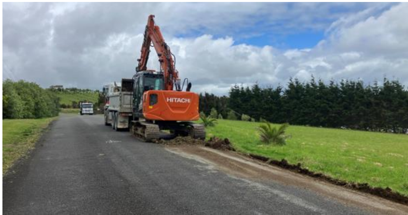
Midgley Road, Mangonui Rehabilitation, starting on site, enabling works.
