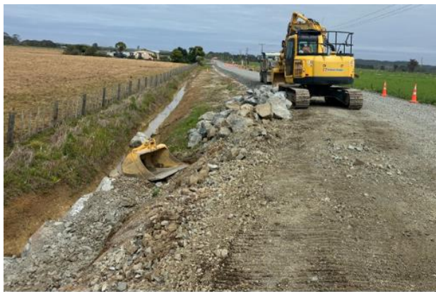
Rockwalling to support shoulders (left) and overlaying of pavement (right)
