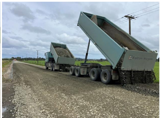
Rockwalling to support shoulders (left) and overlaying of pavement (right)
