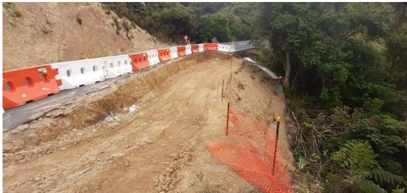
Contract 7/22/150 - FNDC Slip Repairs Suite 01
