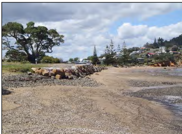
Site Photograph A (north – grouted rock seawall)
