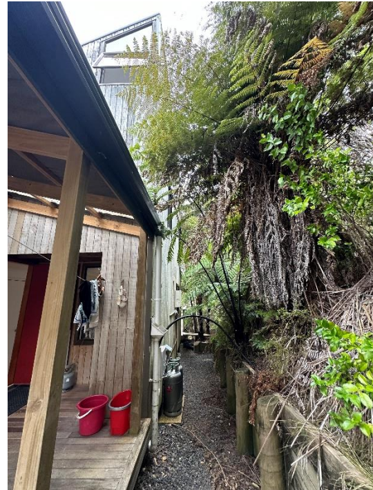
Figure 16: Image showing the steep vegetated slope along the boundary where the setback breach occurs as well as the walkway which can be utilised for maintenance and construction activities.
