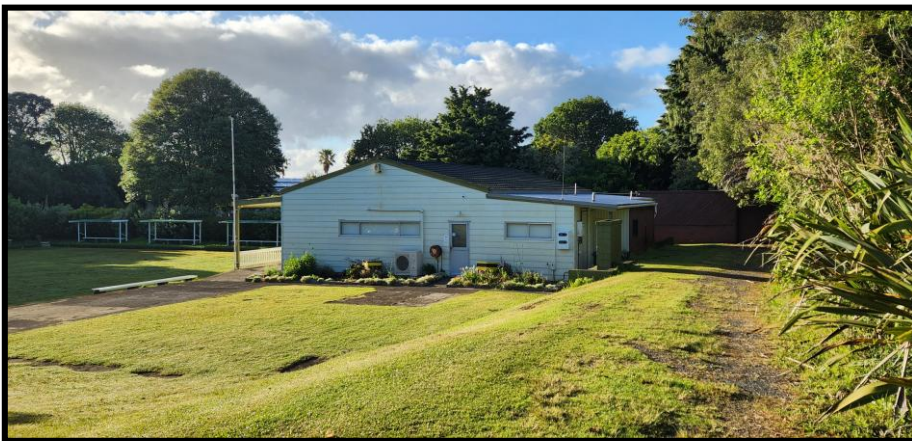
Figure 4 - Existing building and surrounds
