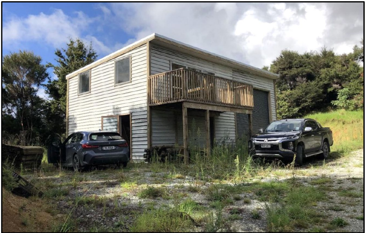
Figure 6: Building within side yard
