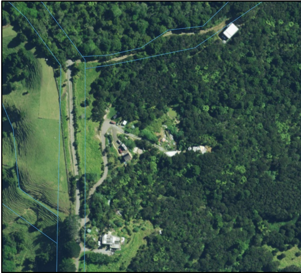
Figure 3: Existing buildings in relation to unconsented building (top right)
