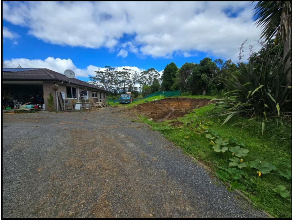
Figure 2: Proposed shed location, with excavations showing extent of shed.
