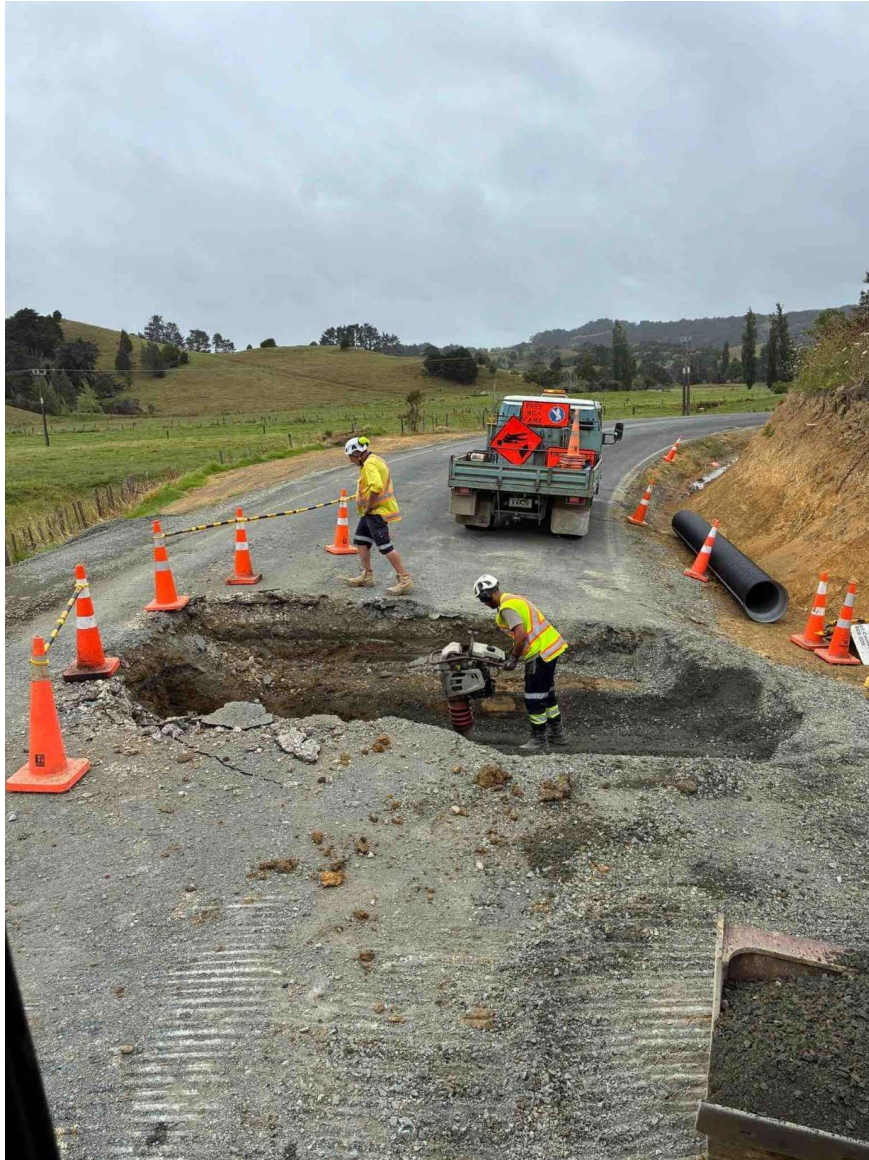
Fairburn Rd Rehab – Drainage replacement in progress
