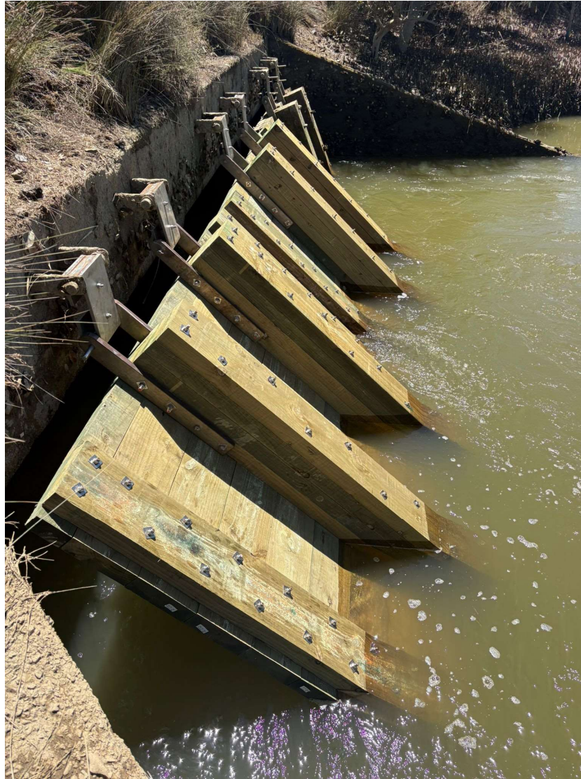
Kohukohu Rd Floodgate Repair
