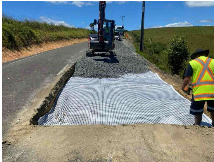
Taupo Bay – Pavement repairs in progress
