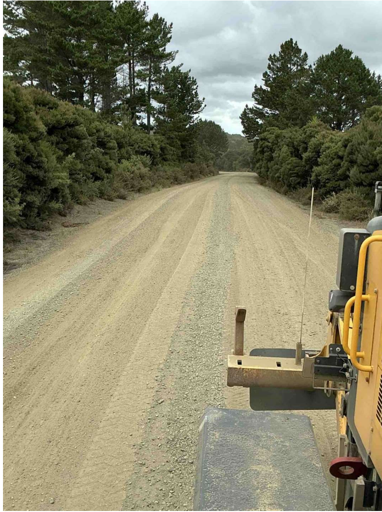
Te Hapua Rd – Maintenance Grading in progress
