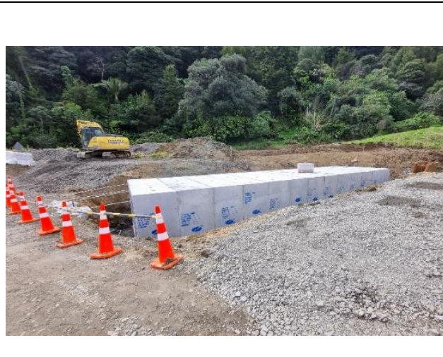
Wekaweka Road J18 Culvert Replacement – ongoing culvert installation
