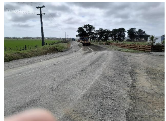
Gills Road Rehabilitation, Water tabling and shoulder strengthening
