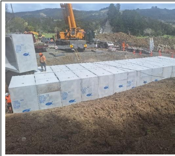
Wekaweka Road J18 Culvert Replacement – ongoing culvert installation
