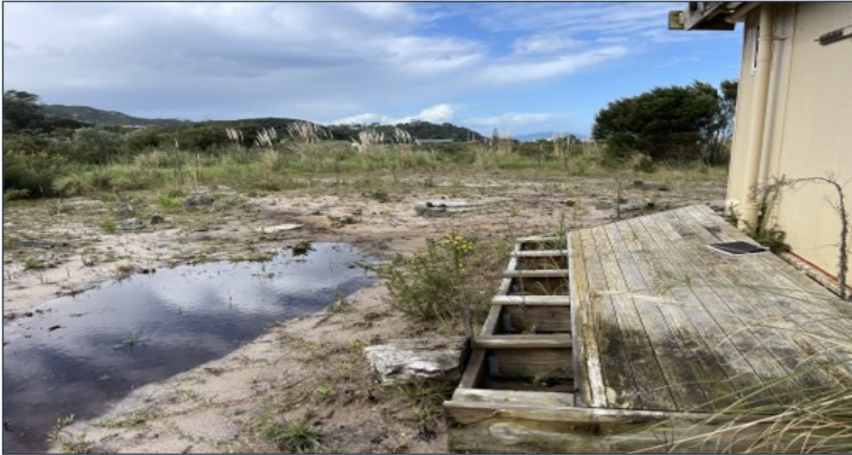
Figure 4: Existing shed and decking
