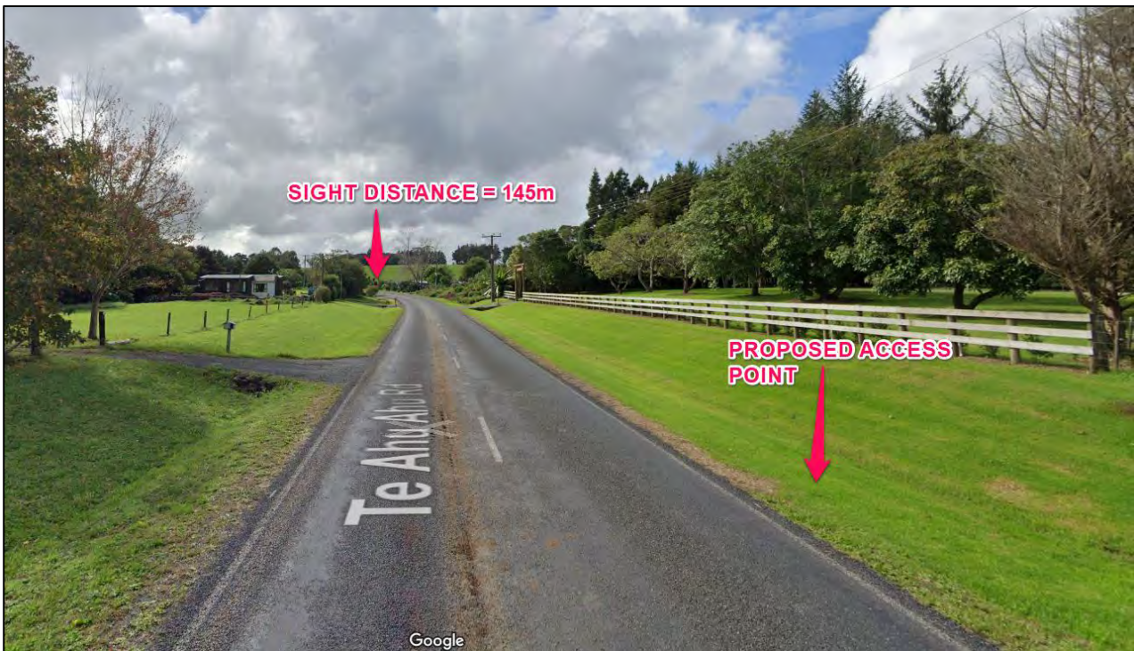
Figure 13: Proposed Access Point on Te Ahu Ahu Road Facing Northeast, ~145m Sight Distance Available.
