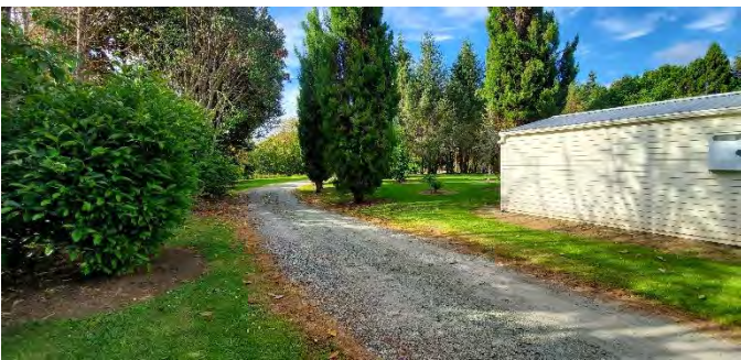
Figure 4: Shed on Lot 1 which creates setback breach. Existing drive to Lot 2.
