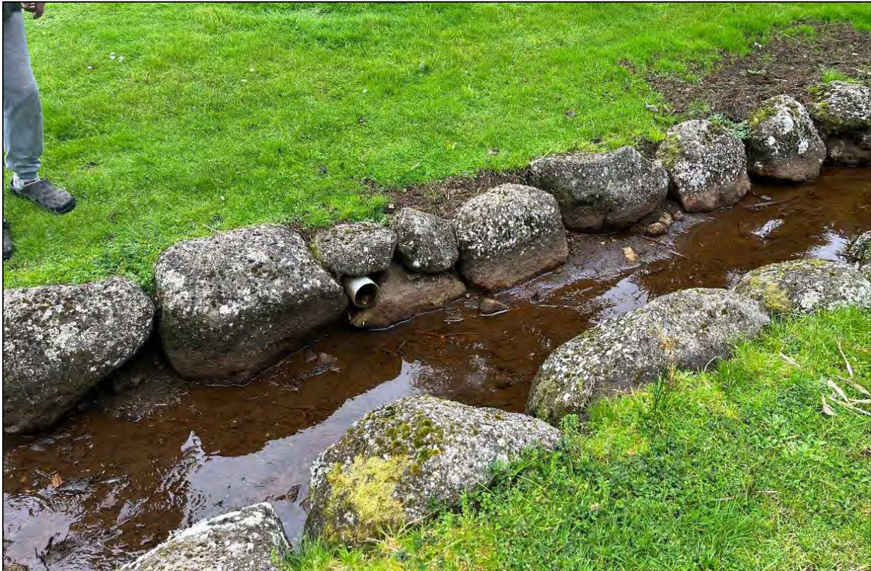
Figure 8: Site Photo Showing Lot 2's Existing Stormwater Discharge Point in Existing Channel.
