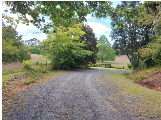
Existing appurtenant right of way, leading into the bend
