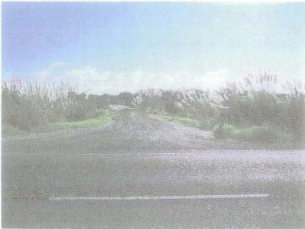
Existing crossing place – note bridge
