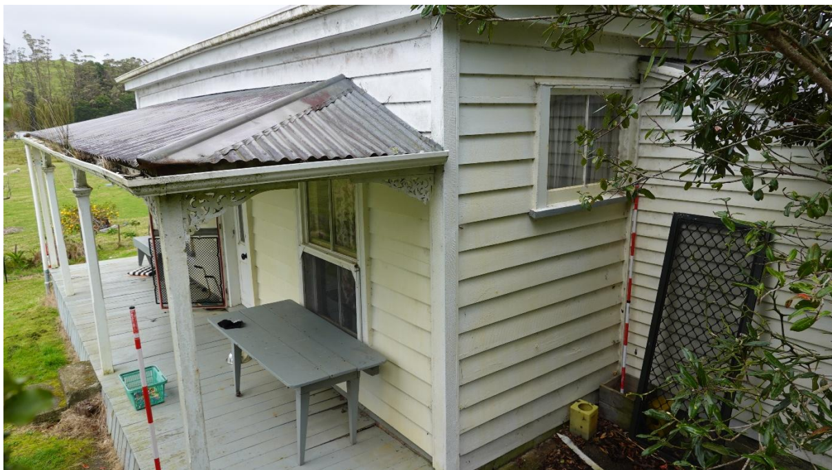
Figure 21. Northeast corner of house. Scale units: 20 cm.
