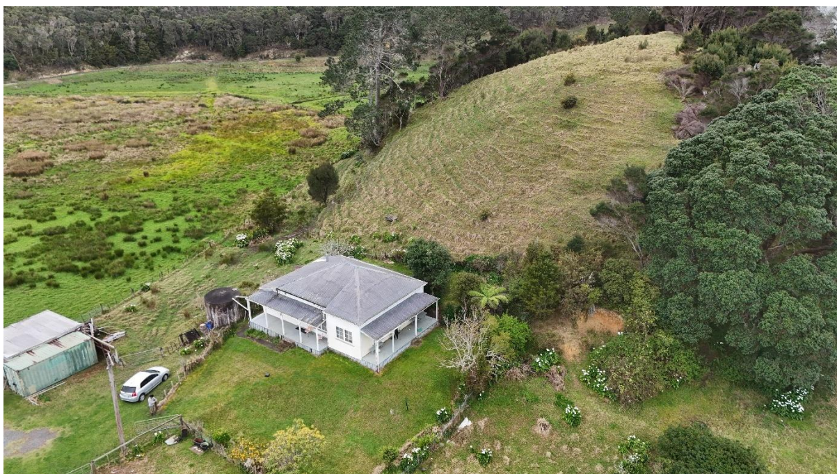
Figure 18. House platform and terraced hill to north.
