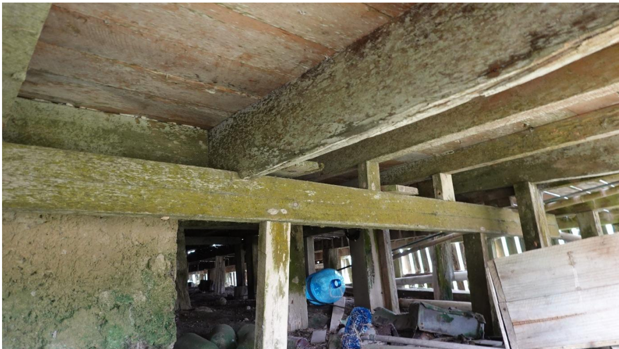
Figure 11. Concrete chimney and timber piles and bearers.
