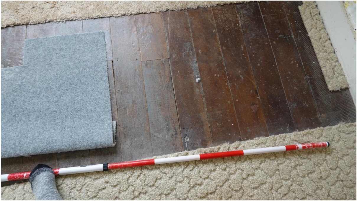
Figure 22. Floorboards in hallway. Probably kauri. Scale units: 20 cm.
