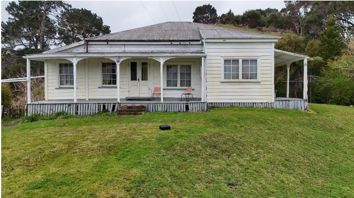
Figure 12. South side of building. Note unusual roof line and shape of right section of building. Scale units: 20 cm.
