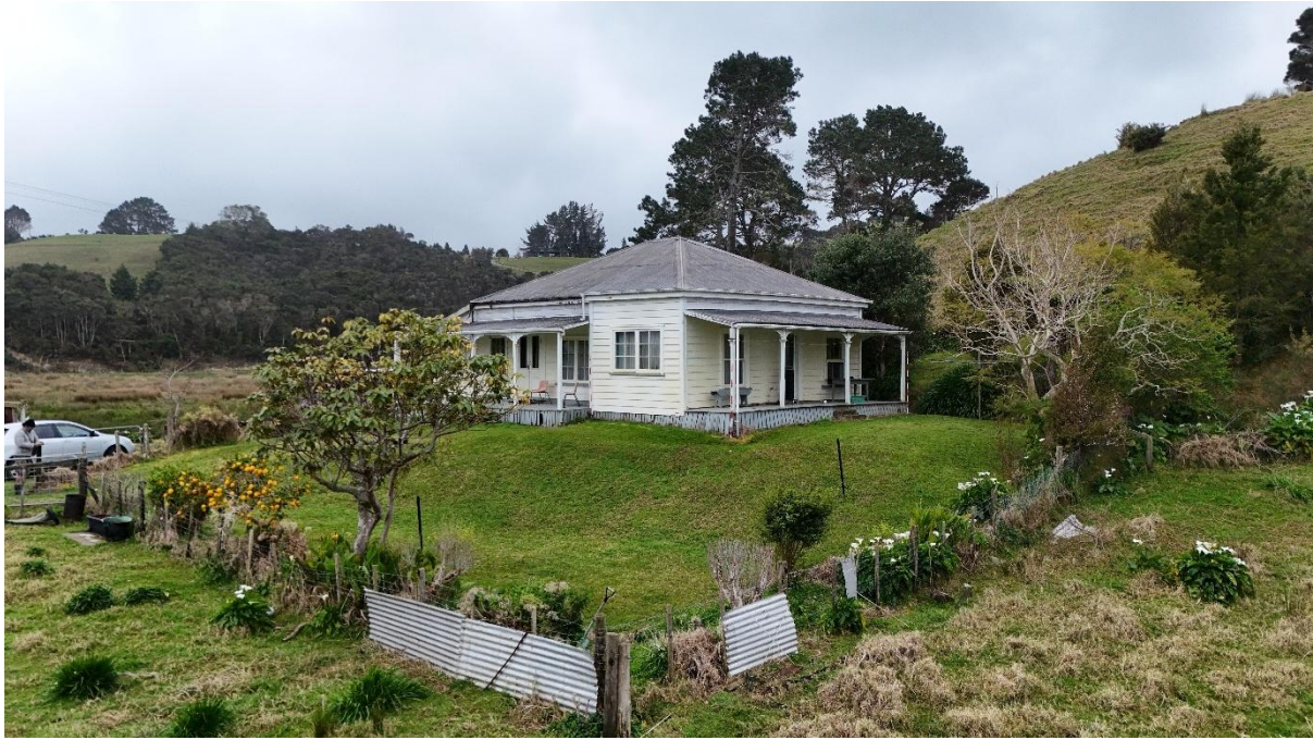
Figure 14. Southeast corner of house. Note raised building platform.
