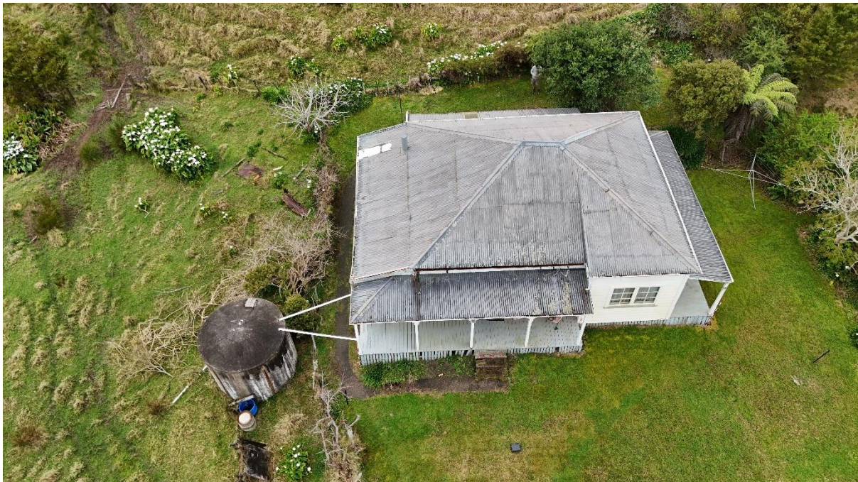
Figure 13. Roof of existing structure. North is top of page.
