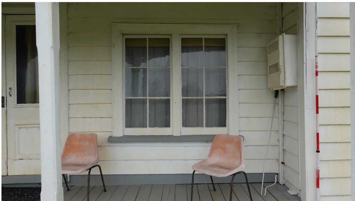
Figure 20. South side veranda. Scale units: 20 cm.
