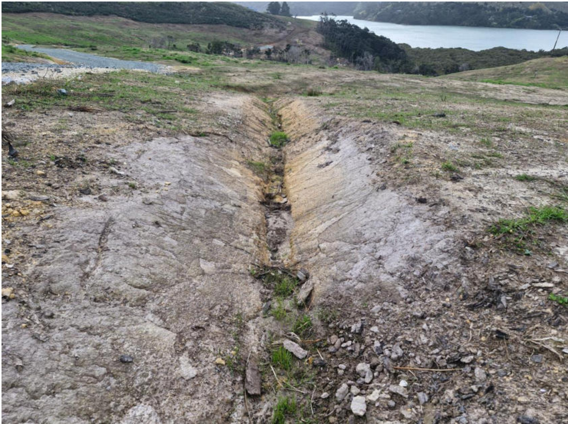
Figure 5: Example of existing formed vee channel for overland flow, from existing culvert near CH140 Road to Vest, displaying less than minor erosion despite lack of vegetation or velocity mitigation.
