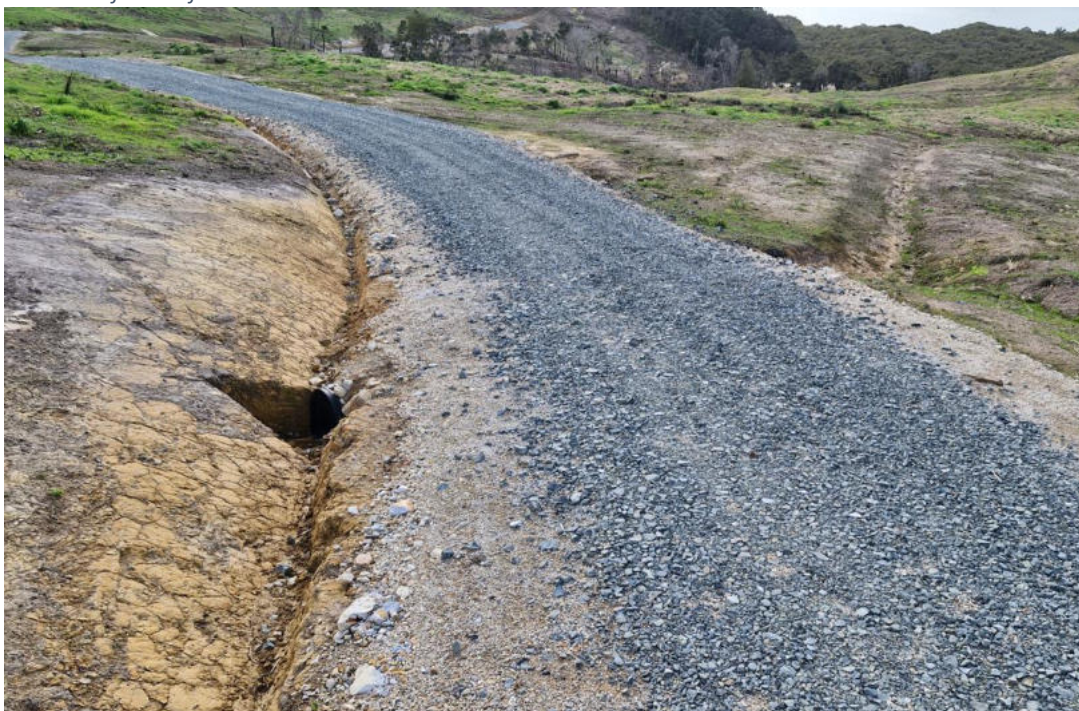
Figure 4: Looking north along existing metal track, showing existing 300Ø PE culvert inlet on left side, draining swale to OLFP on right side, toward CMA.
