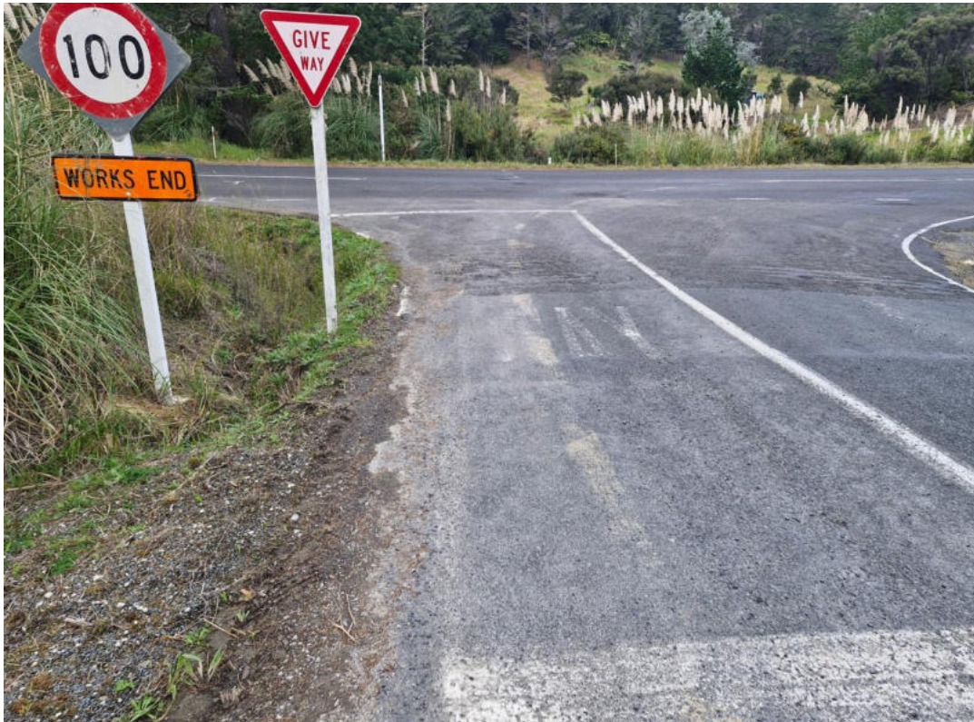
Figure 6: Looking south from Ota Point Road, at its intersection with Wainui Road. Observed weathered edge of seal and road markings.
