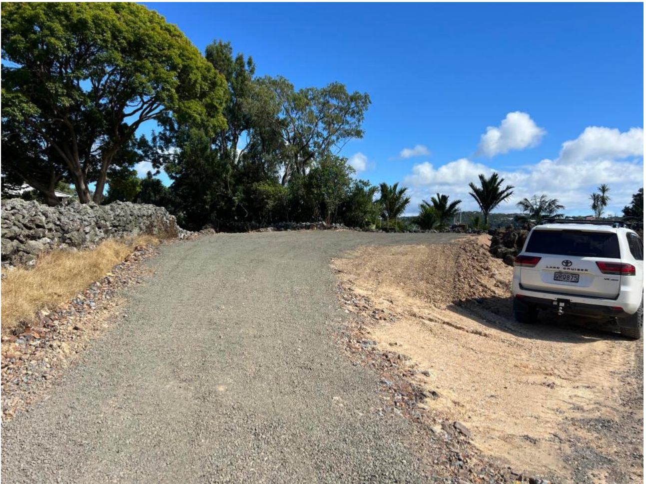
Figure 9. View north over compacted building platform
