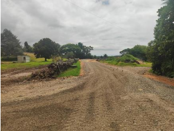
Figure 8 - Easement B recently constructed
