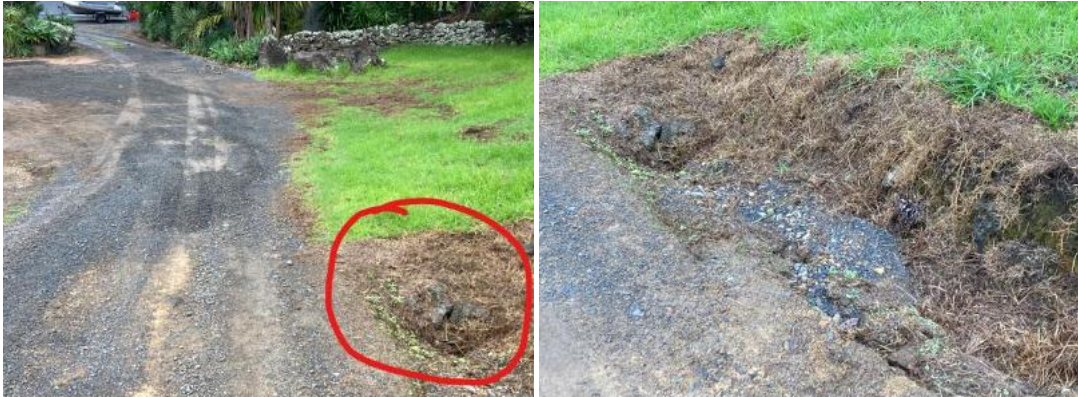
Figure 1: Existing swale outlet (soakage) to fractured basalt, near Ch300m of accessway
