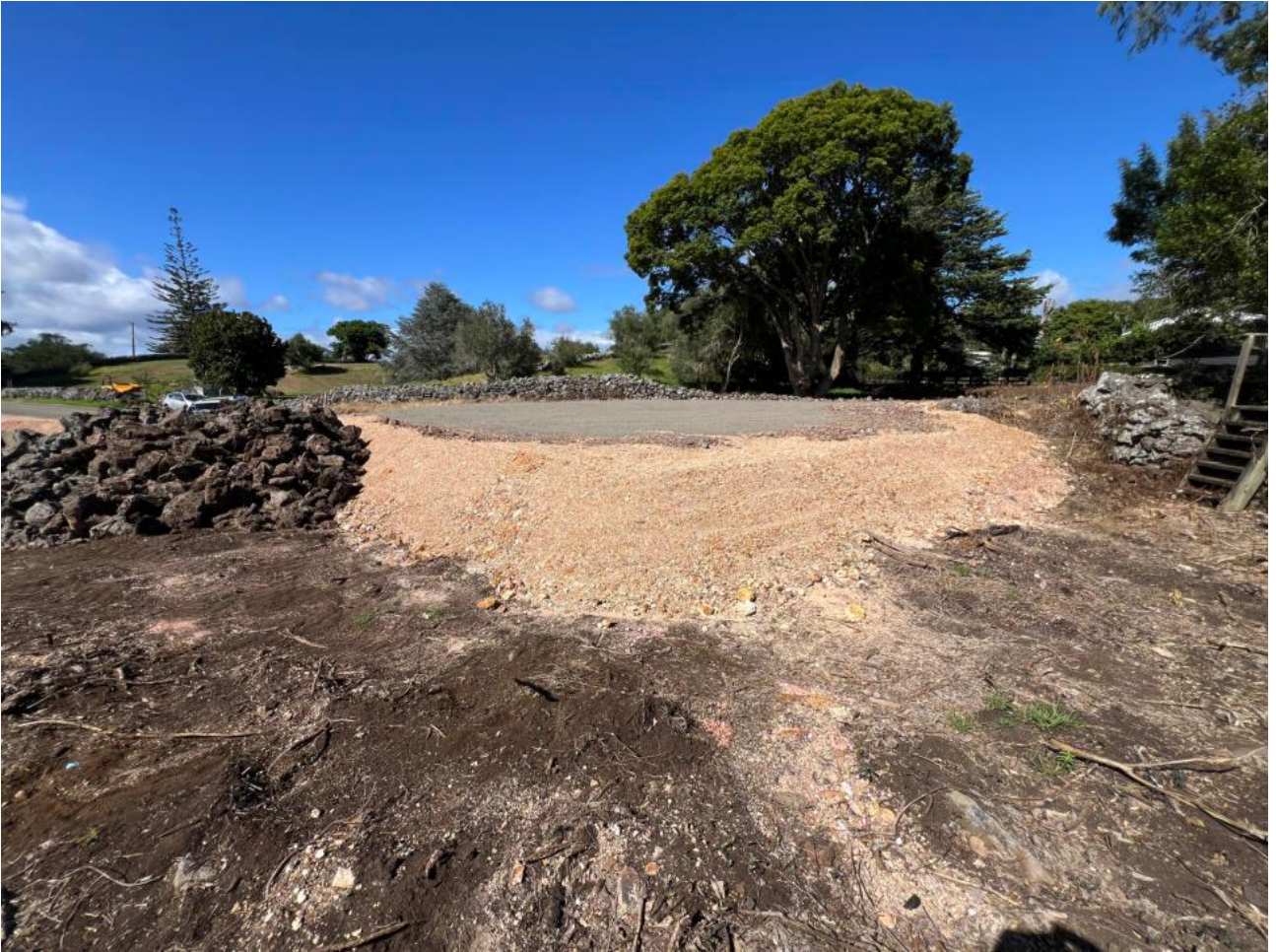
Figure 10. View south over compacted building platform
