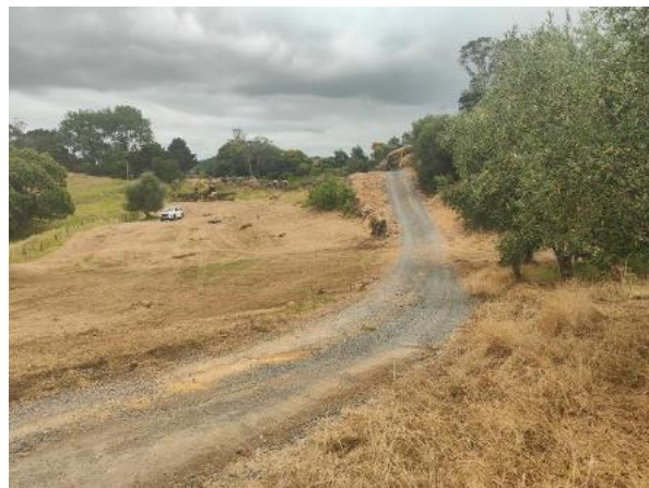
Figure 7 - ROW A driveway with dip proposed to be filled to improve sight visibility on the driveway
