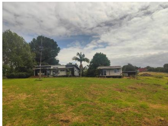
Figure 13 - Dwelling and accessory buildings on Lot 1
