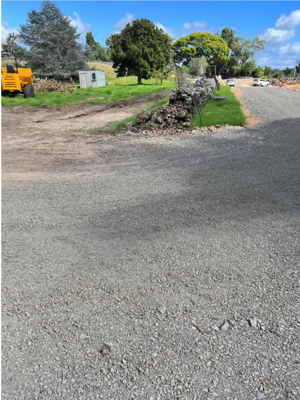
Figure 12. Removed stone wall
