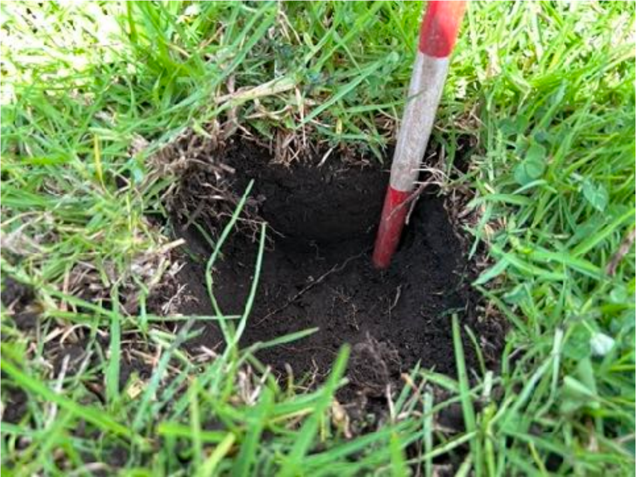
Figure 17. Detail of Test Pit 2.
