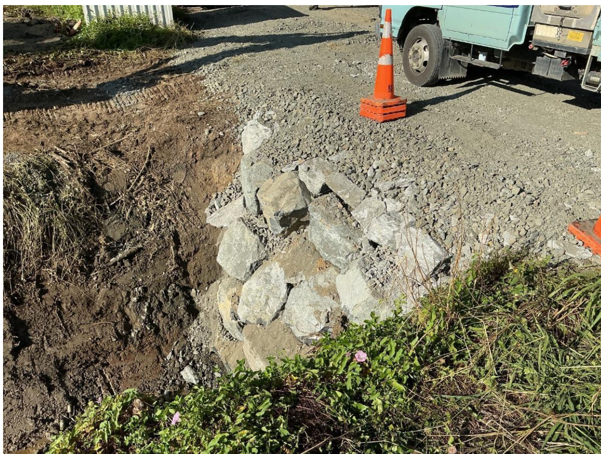
Wells Road Drainage Renewals – Complete
