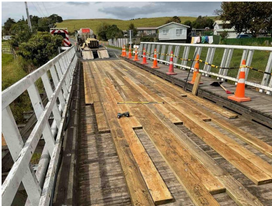
Donald Lane Bridge – Wearing Board Replacement in Progress
