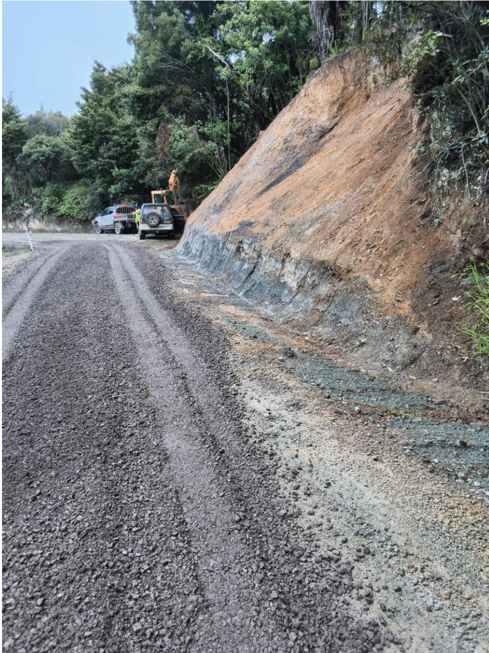
Humpries Rd Slip Retreat - Complete
